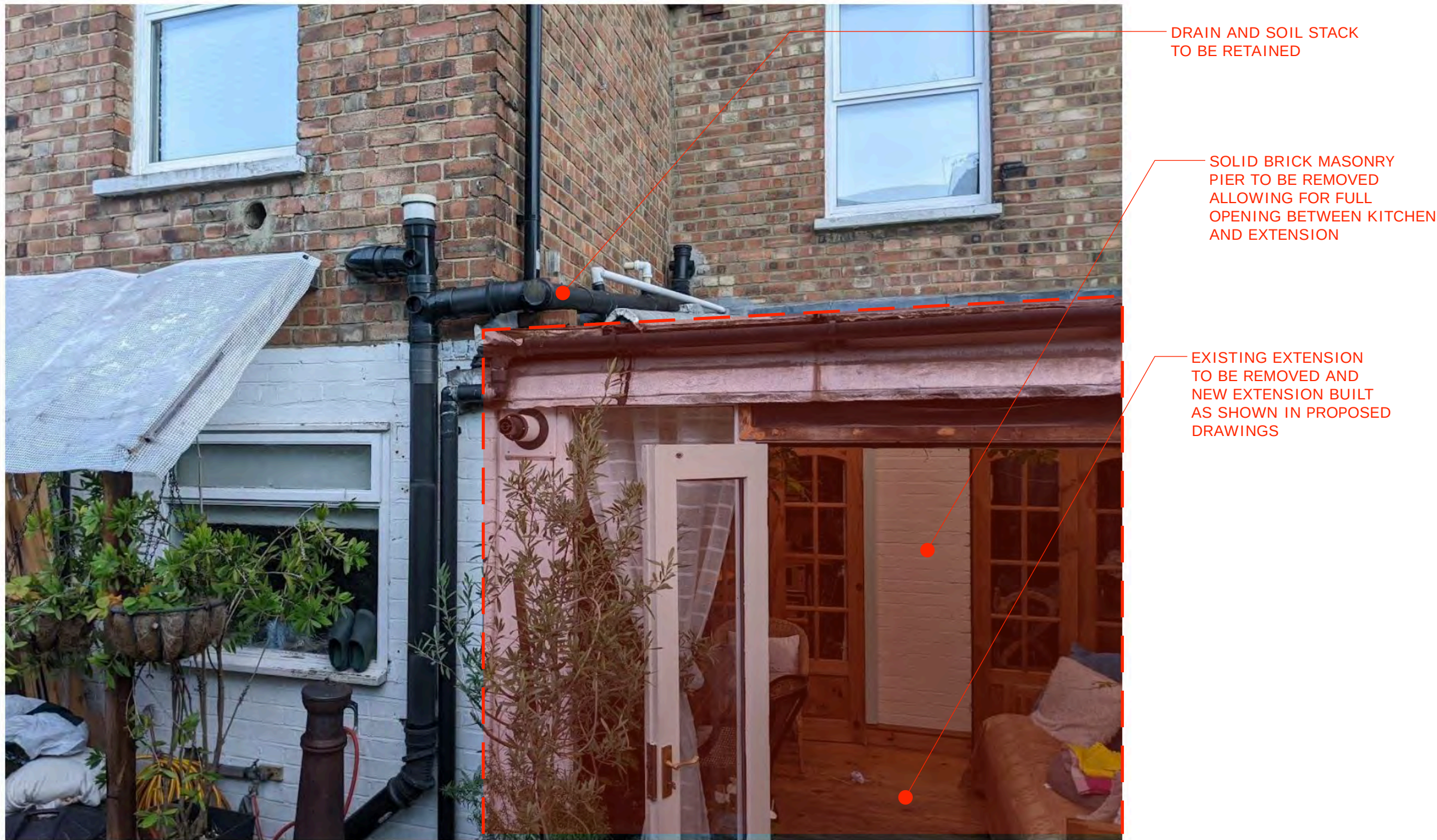
VIEW FROM GARDEN AT EXISTING EXTENSION
