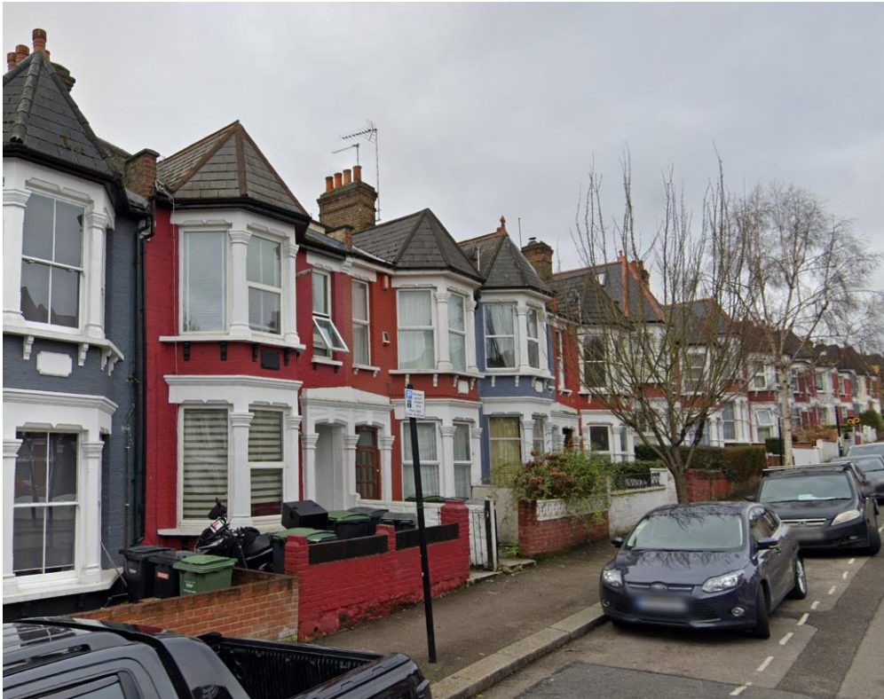
Figure 4: 70 Duckett Road - Street View - Photo showing terrace housing
