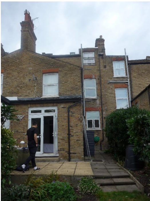
Rear view of no. 14 Nelson Road
