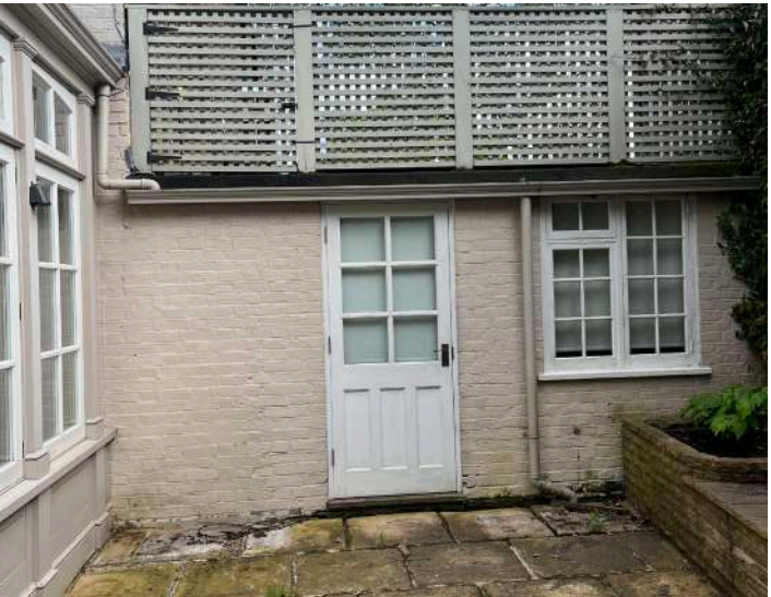
4. View of rear garage
