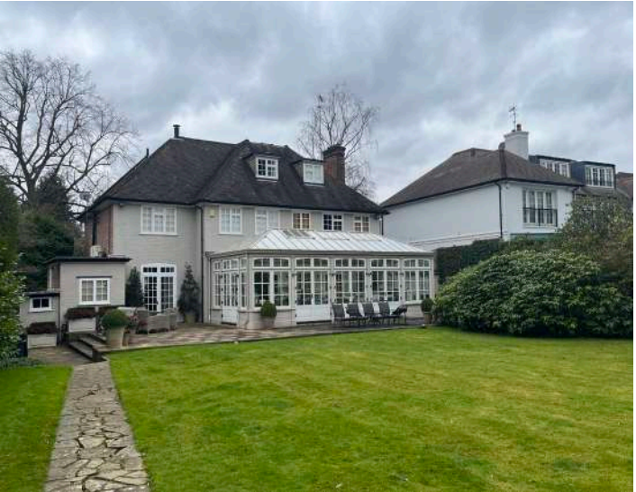
2. View of rear elevation
