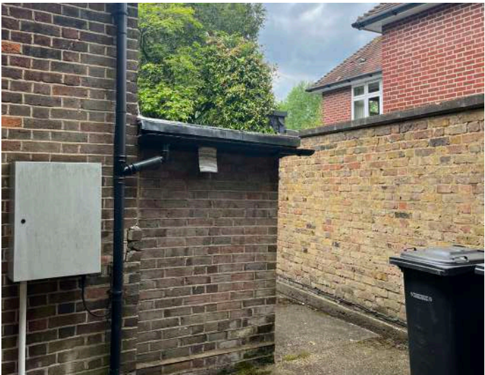
5. Flank facade brickwork
