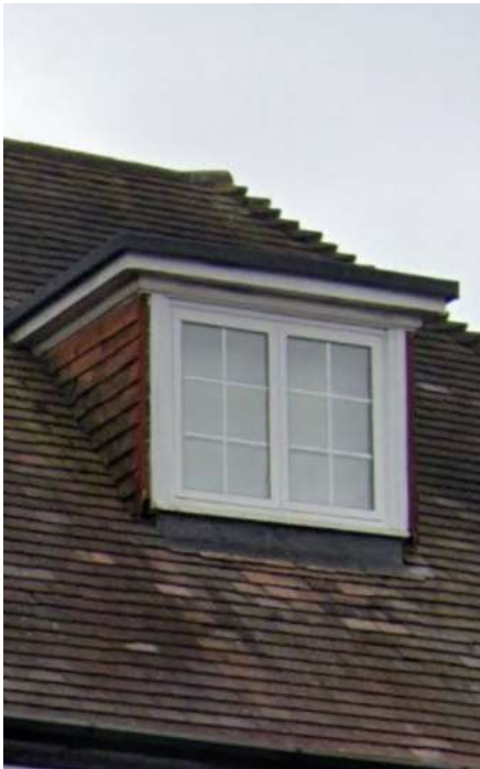
Clay roof tiles, dormer windows and timber eave details
