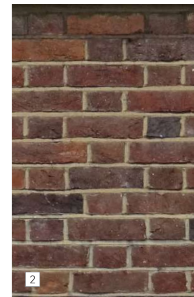
Brickwork to match existing
