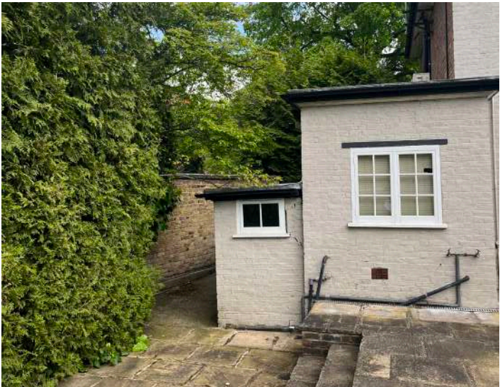
3. View of one-storey rear elevation
