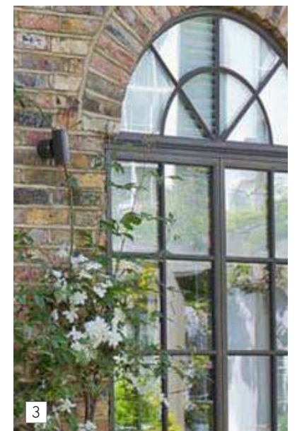
Metal framed glass doors
