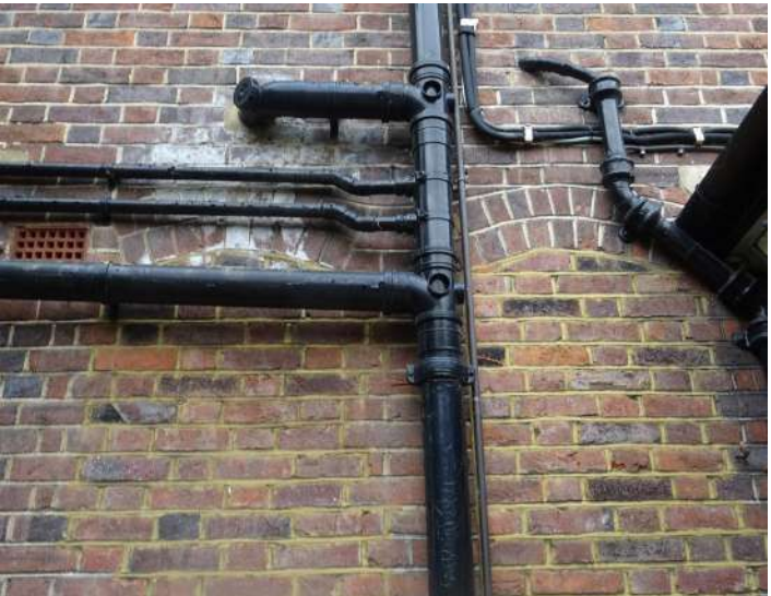
6. Flank facade brickwork
