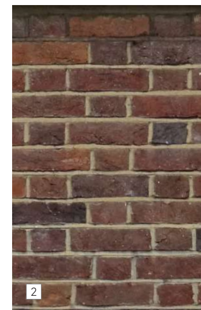
Brickwork to match existing
