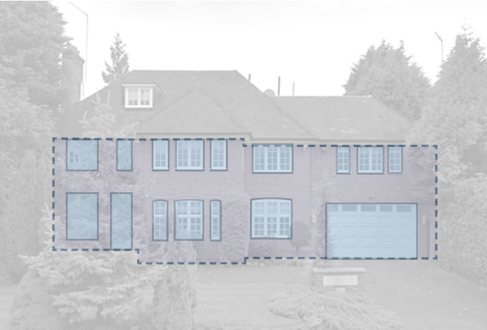
F 33 Sheldon Avenue Openings percentage (excluding roof): 38%
