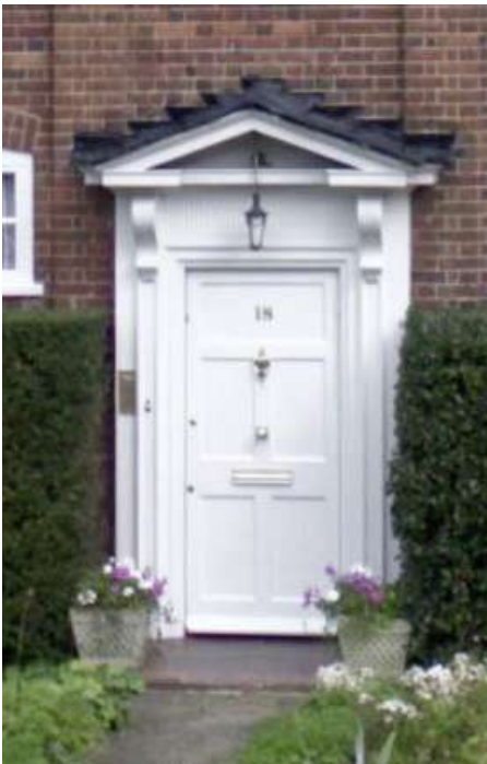
Painted timber door surrounds
