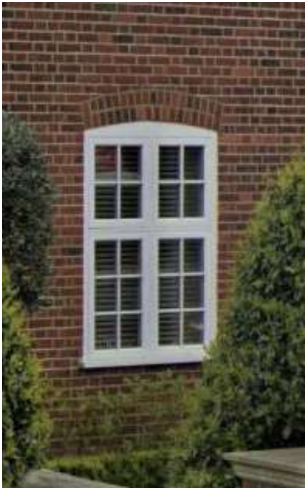
Timber framed windows, set to the outer face of the walls
