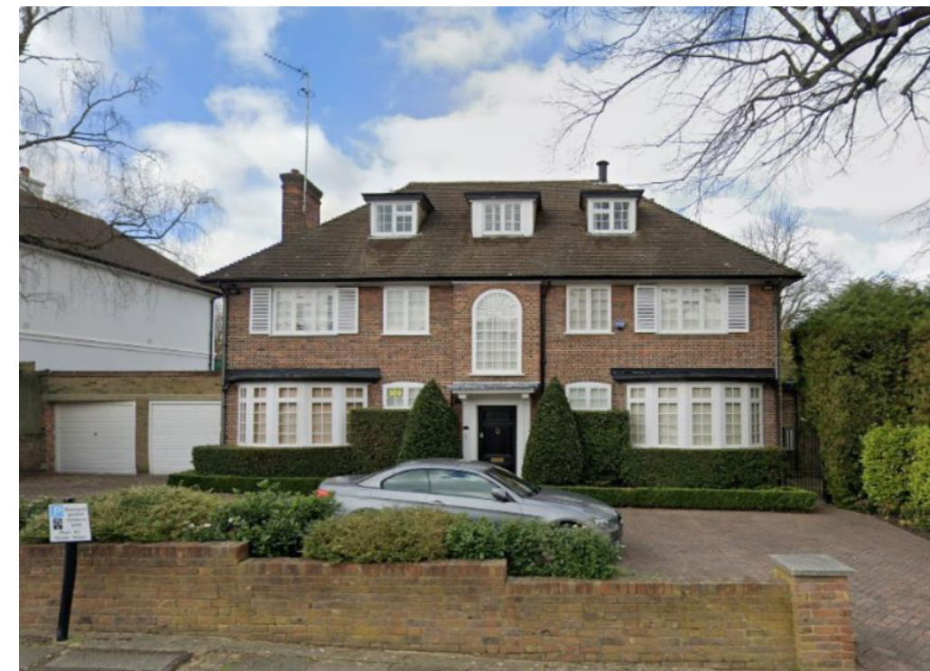
Figure 4. View of the existing property front elevation.
