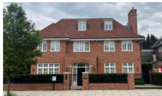
Figures 18 & 19: The pre existing house at no.28 Sheldon Avenue (top) and the replacement building (bottom).
