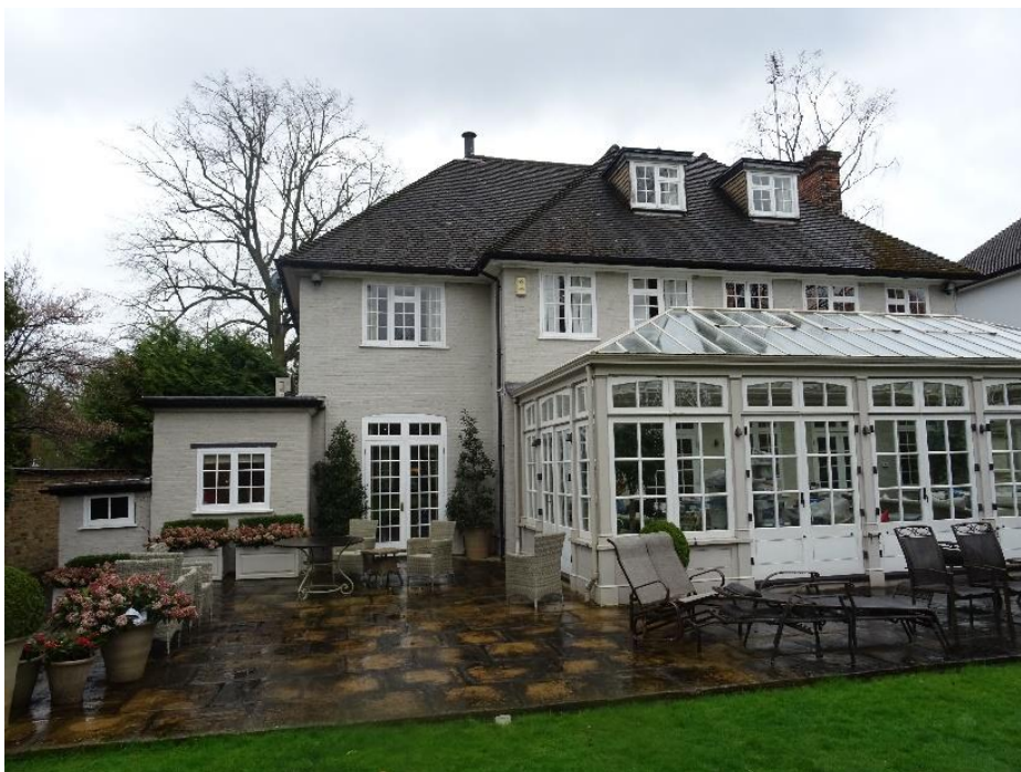
Figure 11: The rear façade of the house.
