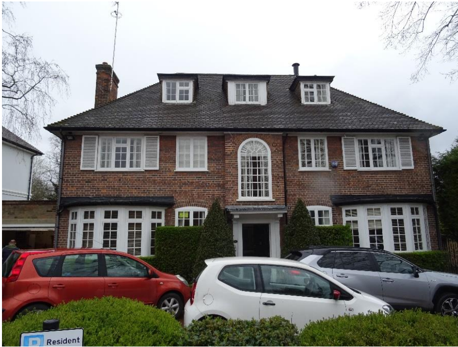
Figure 10: The front façade of the house.
