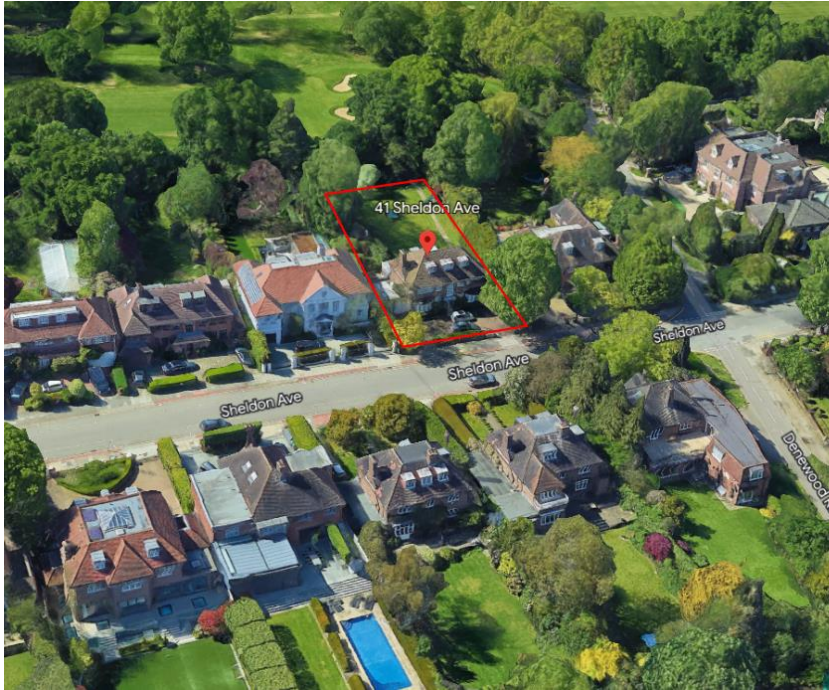
Figure 2: Site Photo (©Google Maps, 2022)
