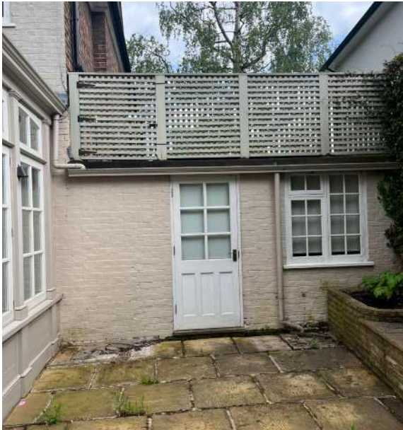
View 5 - Rear of garage side extension
