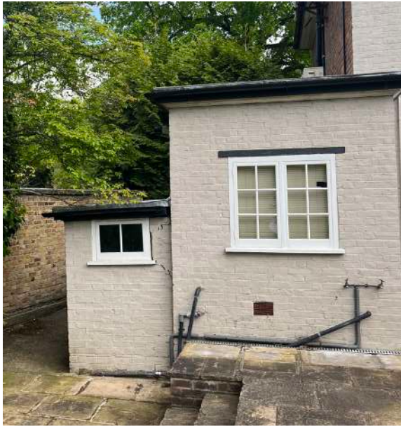
View 6 - View of side extension
