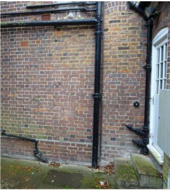
View 9 - View of north elevation
