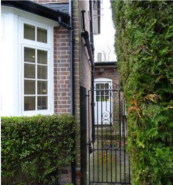
View 2 - Passage through side of building
