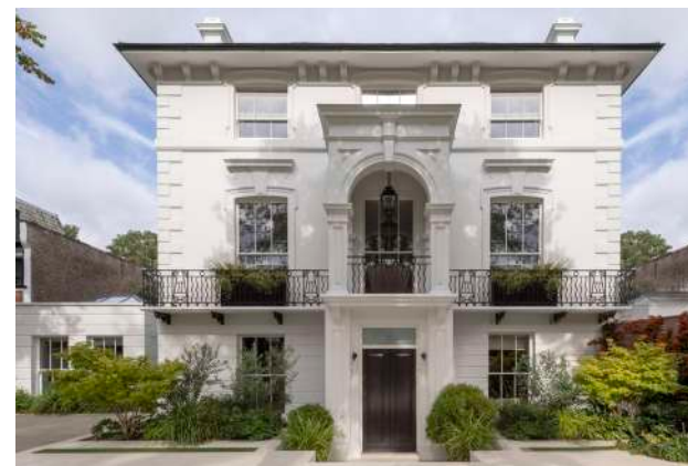
Langford Place (Grade II listed), 5,927sqft St John's Wood Conservation Area
