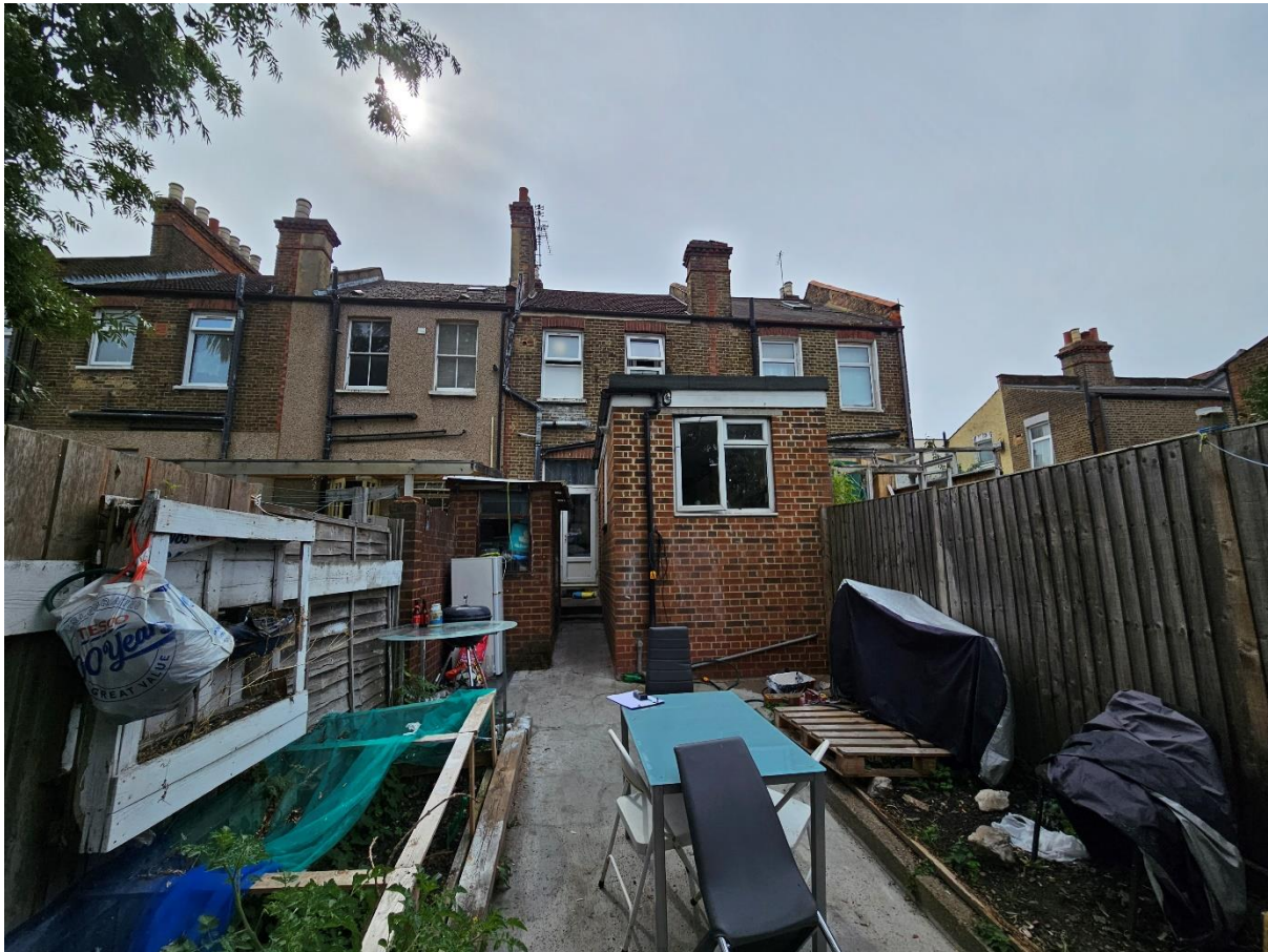
Rear Elevation Photo
