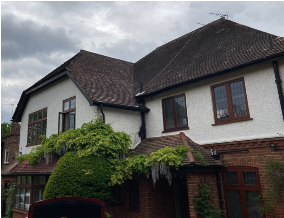
11 and 11A View Road – Existing
