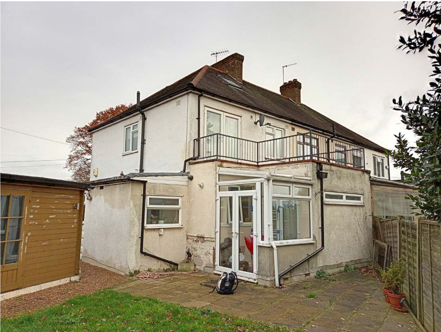
fig. 01 - Rear view of the existing property.
