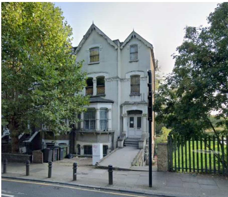
Google Street View Image September 2020. Note the presence of multiple refuse bins suggesting that the building contains more than one dwelling.
