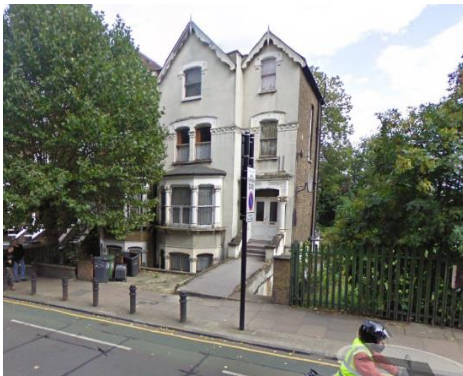
Google Street View Image September 2011. Note the presence of multiple refuse bins suggesting that the building contains more than one dwelling.
