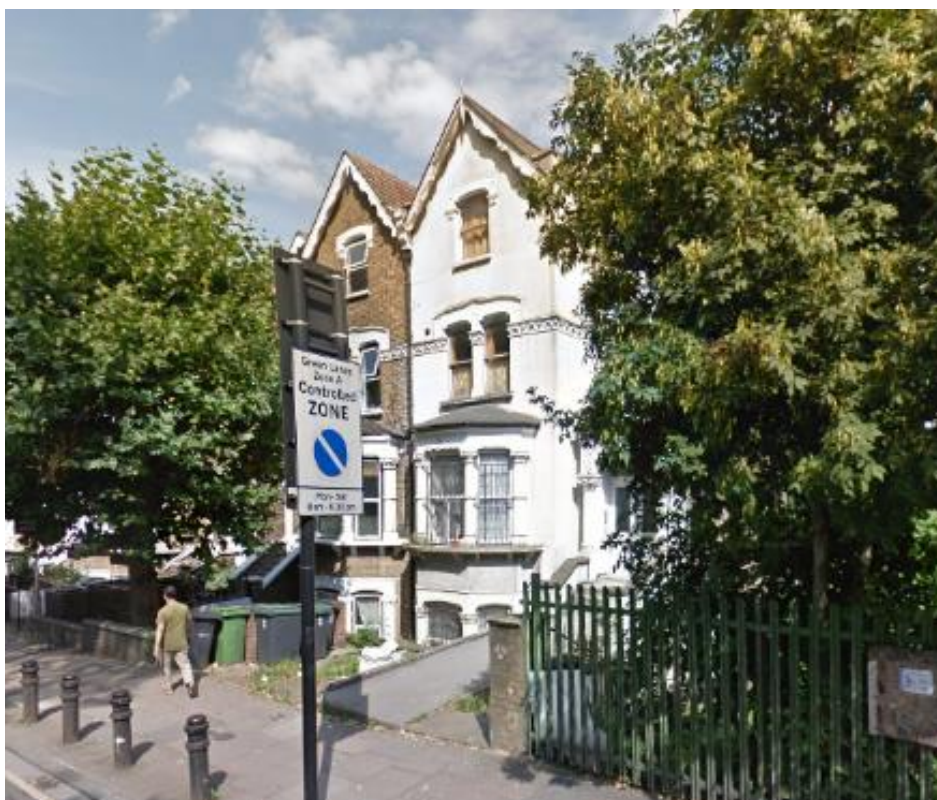
Google Street View Image August 2017. Note the presence of multiple refuse bins suggesting that the building contains more than one dwelling.
