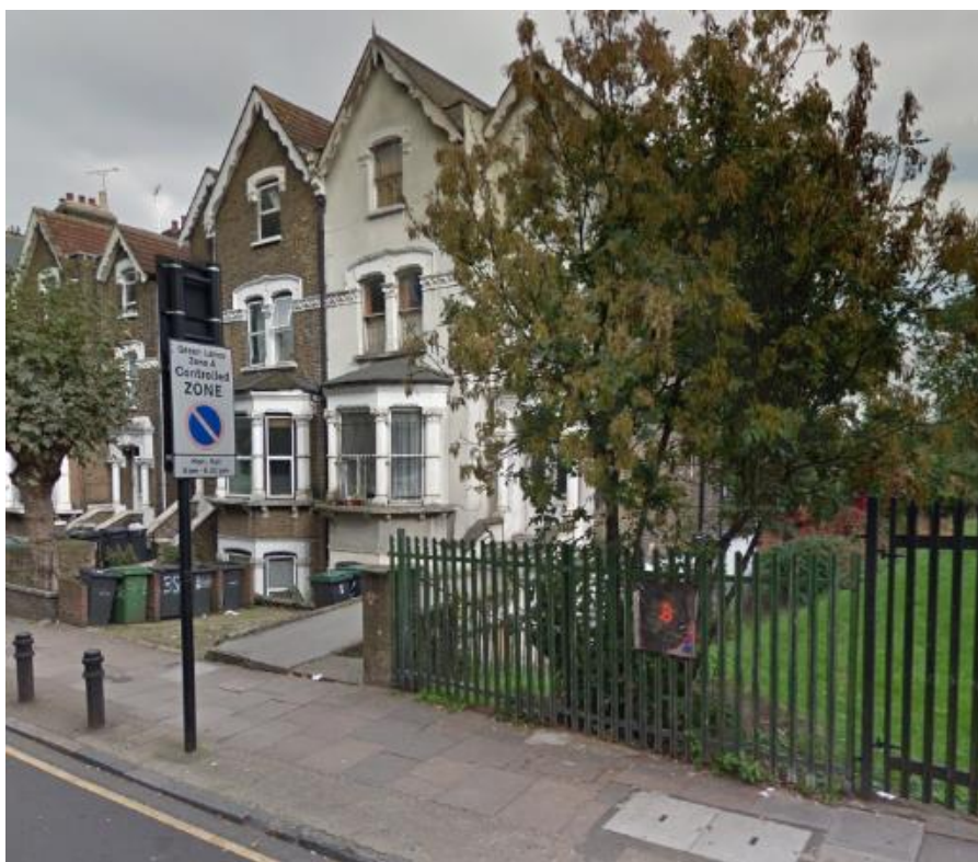
Google Street View Image October 2015. Note the presence of multiple refuse bins suggesting that the building contains more than one dwelling.
