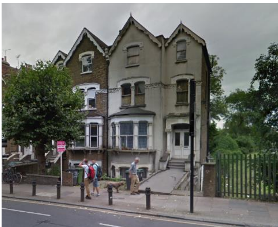
Google Street View Image August 2016. Note the presence of multiple refuse bins suggesting that the building contains more than one dwelling.
