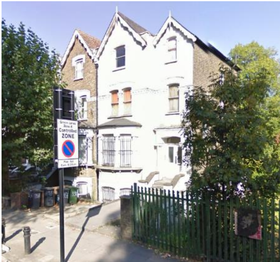
Google Street View Image September 2009. Note the presence of multiple refuse bins suggesting that the building contains more than one dwelling.
