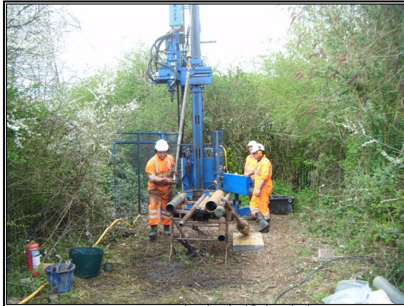
Plate 1. Drilling of BH7
