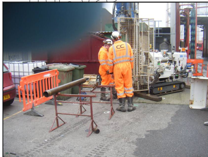
Plate 2. Drilling set up at BH12-03, south of the bus wash.
