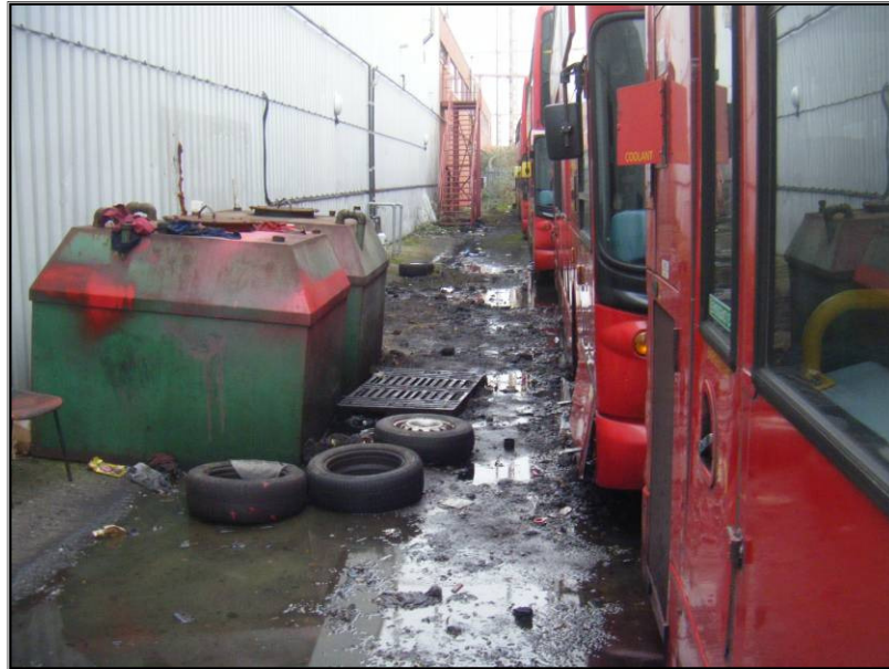
Plate 5. Un-bunded waste tanks located behind workshop. Visible contamination on ground surface throughout the area.
