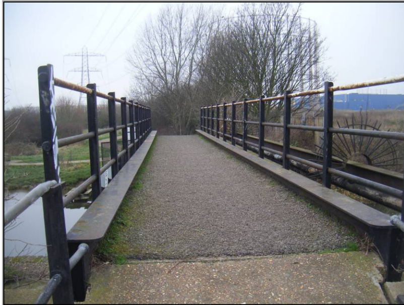
Plate 7. Footbridge across River Lea Navigation Canal, looking west.
