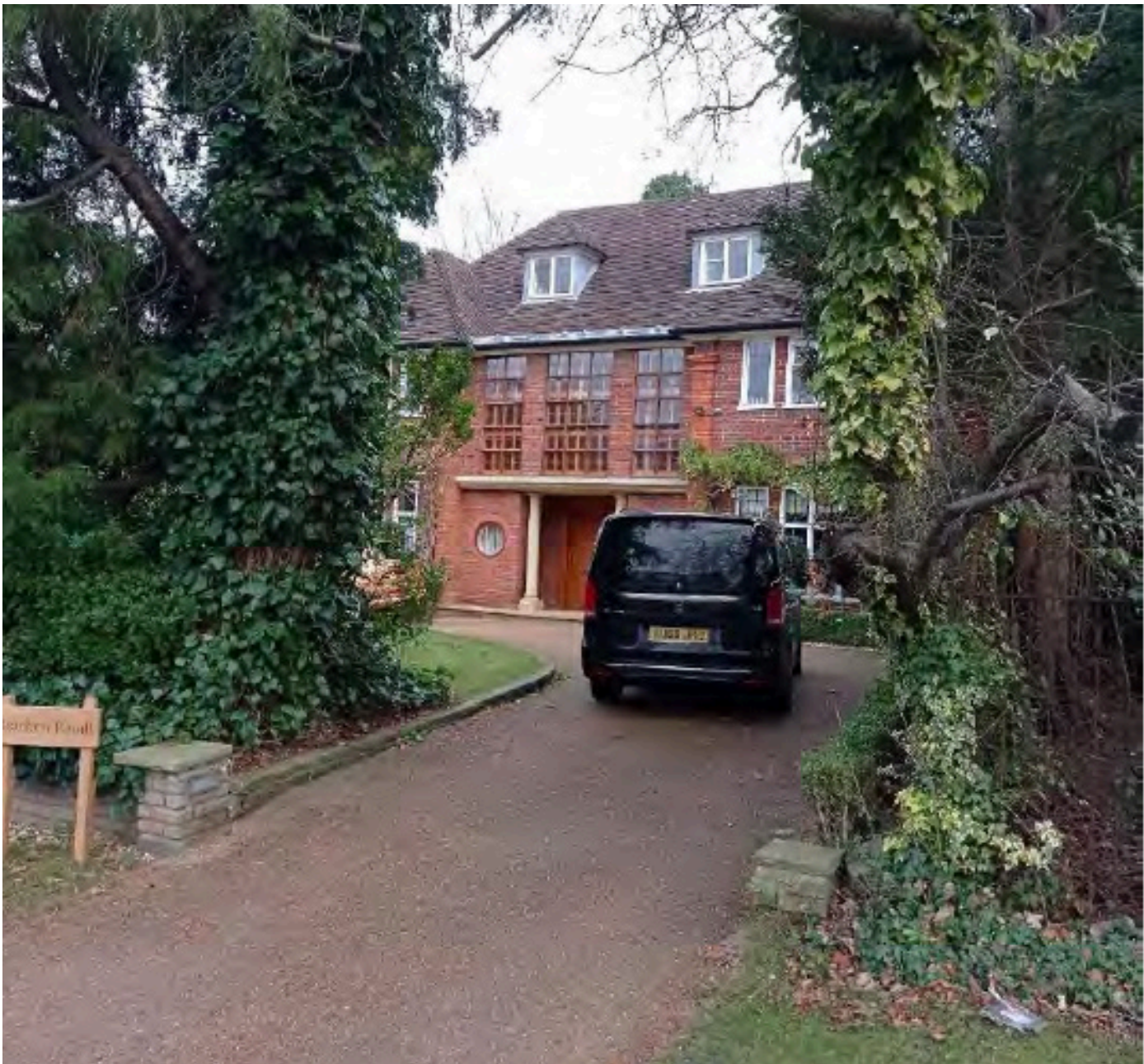
View of existing front elevation of Bracken Knoll from the main private access road.
