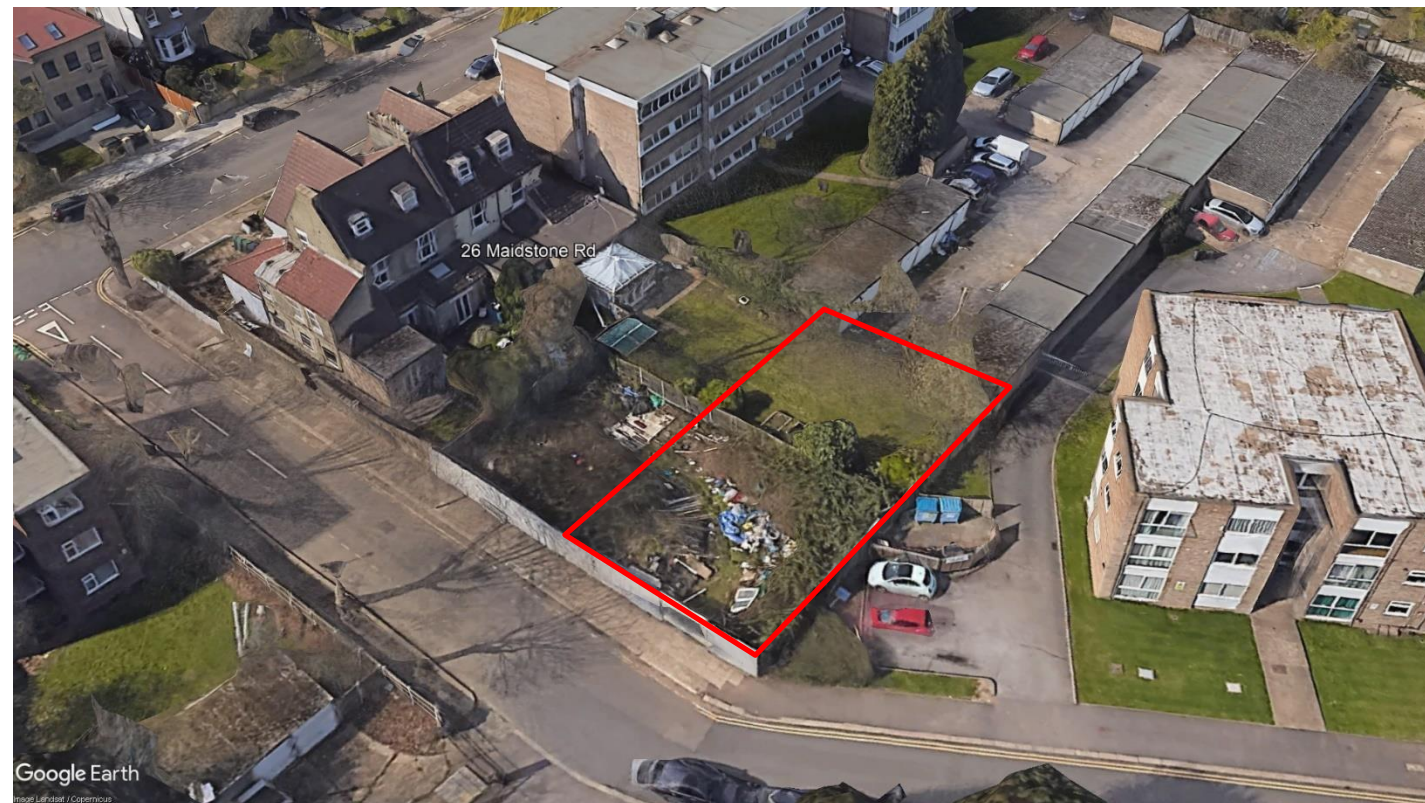
Aerial view of the site as existing, taken on June 03, 2022, from Google Earth.
