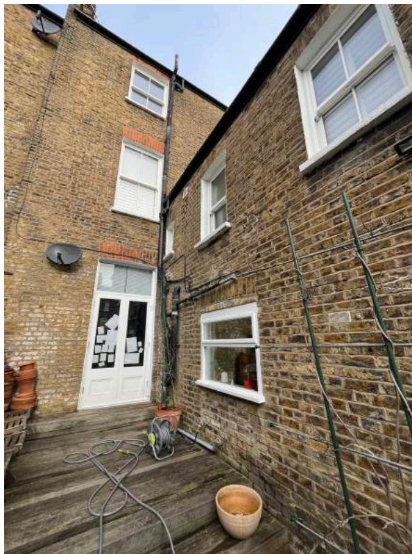
View of existing rear wall and flank wall of closet wing
