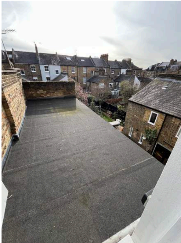
View of existing flat roof of closet wing
