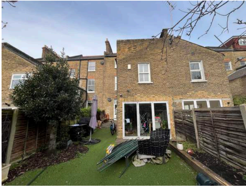
View of existing rear closet wing
