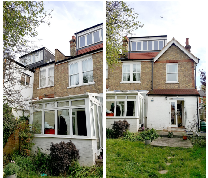
Looking towards neighbour 127 Dukes Avenue closet wing & existing rear elevation to 125 Dukes Avenue
