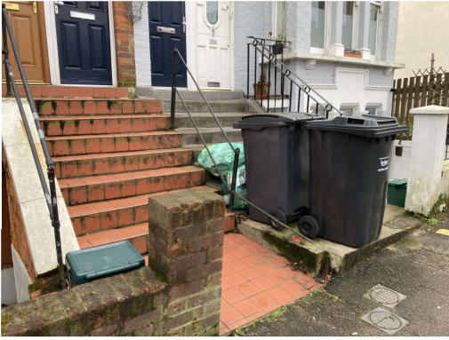
04 VIEW OF COMMUNAL ENTRANCE STEPS FROM THE STREET Existing Site Photograph 04
