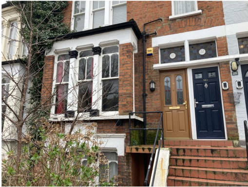
05 VIEW OF RAISED GROUND FLOOR FRONT ELEVATION FROM THE BOTTOM OF THE COMMUNAL STEPS Existing Site Photograph 05
