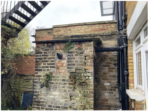
13 VIEW OF BRICK SHED TO BE RETAINED BUT BRICKWORK REPAIRED AND REPOINTED AND EXTERNAL PIPEWORK TO BE SIMPLIFIED Existing Site Photograph 13
