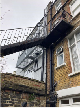
12 VIEW OF REAR GARDEN STEEL STAIRCASE PROVIDING ACCESS NO. 31A FLAT'S REAR GARDEN Existing Site Photograph 12
