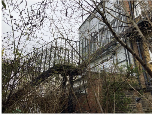
11 VIEW OF REAR GARDEN STEEL STAIRCASE PROVIDING ACCESS NO. 31A FLAT'S REAR GARDEN Existing Site Photograph 11
