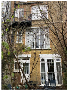
15 VIEW OF REAR ELEVATION OF NO. 31 LOWER AND RAISED GROUND FLOOR WINDOWS AND EXTERNAL DOORS Existing Site Photograph 15
