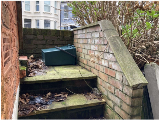
09 VIEW OF STEPS UP TO STREET FROM THE LOWER GROUND GARDEN AREA Existing Site Photograph 09
