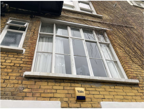
16 VIEW OF REAR ELEVATION OF NO. 31 RAISED GROUND FLOOR WINDOWS Existing Site Photograph 16
