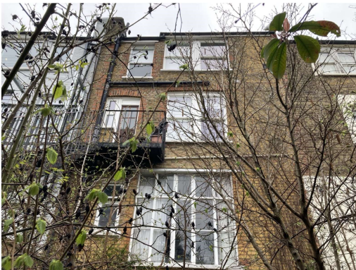
14 VIEW OF REAR ELEVATION OF NO. 31 RAISED GROUND FLOOR WINDOWS AND 31A ABOVE FROM REAR GARDEN Existing Site Photograph 14
