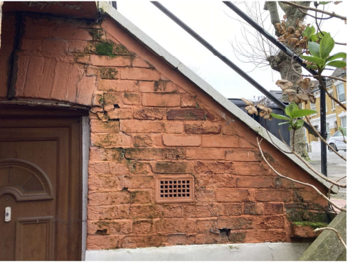
08 VIEW OF LOWER GROUND FLOOR EXTERNAL DOOR AND WALL TO SIDE OF COMMUNAL STEPS Existing Site Photograph 08
