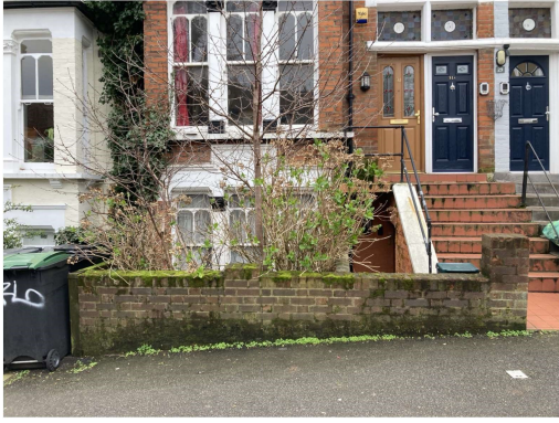
06 VIEW OF FRONT GARDEN WALL FROM THE STREET Existing Site Photograph 06
