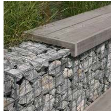
3. Gabion terracing/ retaining walls
