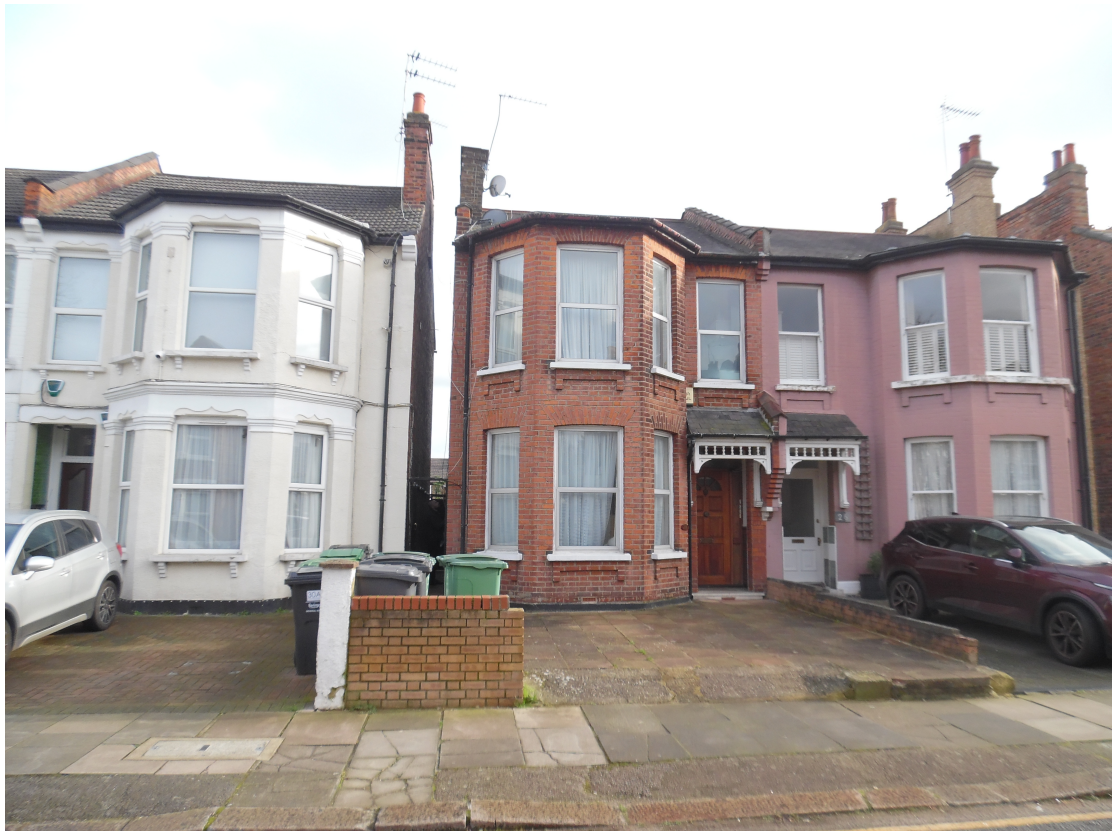
Front view from Palmerston Road
