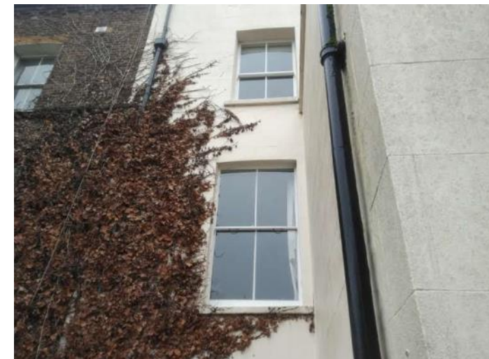
Figure 5.36: Showing the raised ground and first floor windows on the rear elevation of the main building.
