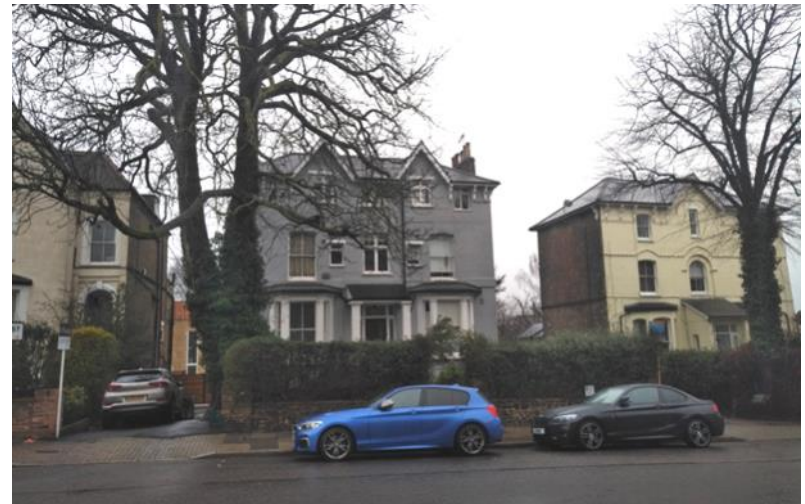
Figure 6.3: Showing 19 Haringey Park in the centre.
