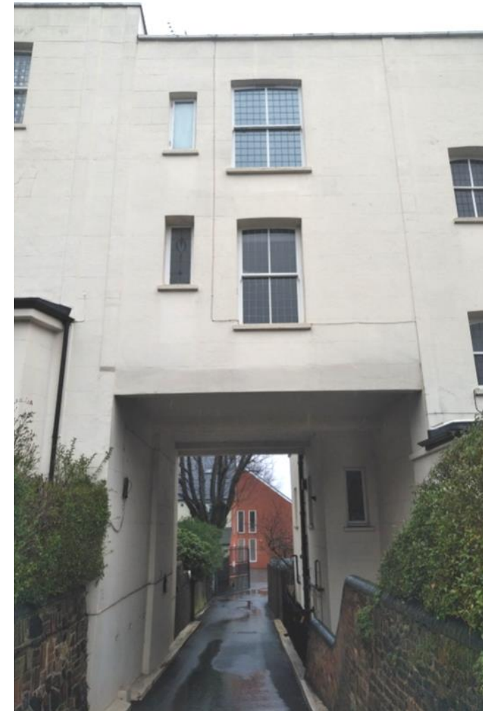
Figure 5.18: Showing the Infill Extension and carriageway.
