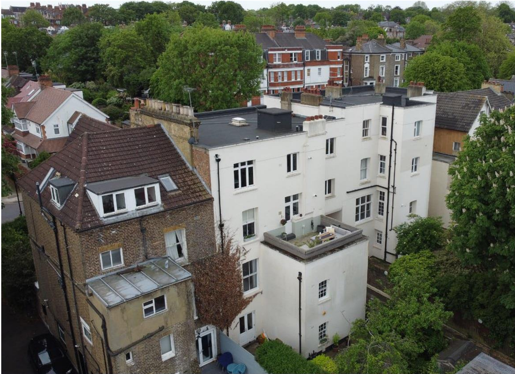
Figure 5.25: Showing the rear elevation of Nos. 16-17 and their rear extensions (Source: Cooke Fawcett Architects DAS).
