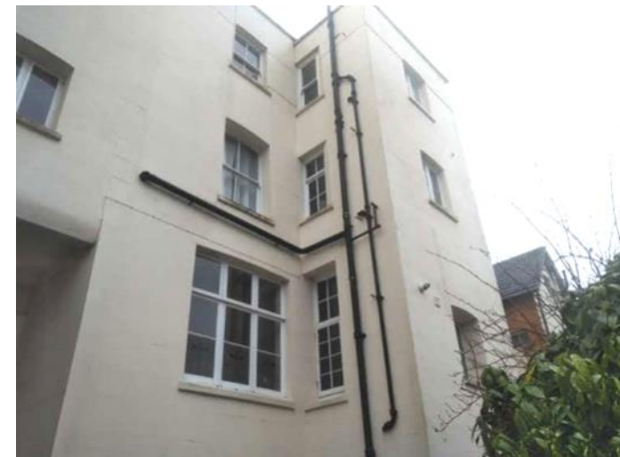
Figure 5.30: Showing the eastern side of the rear elevation at raised ground floor to second floor levels.
