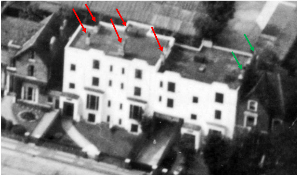
Figure 5.5: By 1938 Harcourt House/Mansions was in existence and we can see a flat roof in this photograph. We can also see flat faux gables along the parapet line, a detail missing today (Source: Britain from Above). We have marked in red the historic chimneys retained on No. 16 at this time. We have also marked in green the historic chimneys retained on No. 17 at that time.
