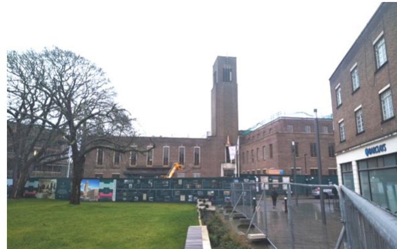
Figure 6.12: Former Hornsey Town Hall.
