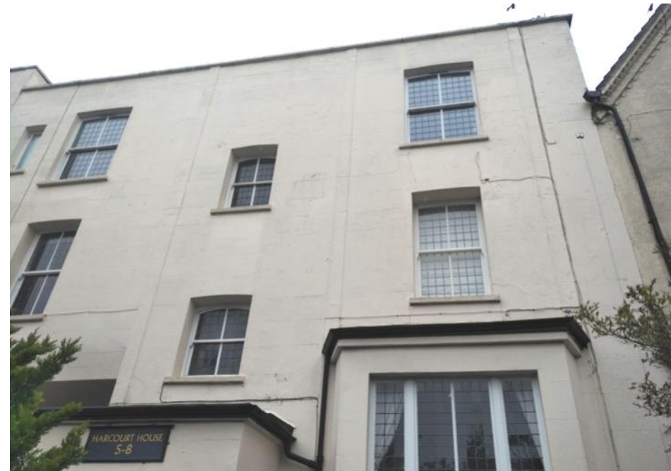
Figure 5.24: Showing No 17 Haringey Park at first and second floor levels.
