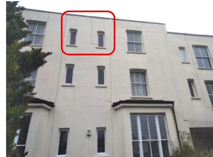
Figure 5.16: Showing No. 16 Haringey Park at first and second floor levels. The area of vertical extension at second floor level is marked in red.
