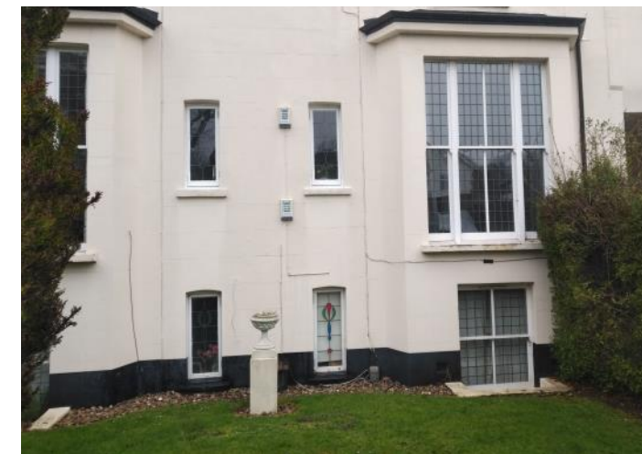
Figure 5.13: Showing part of the front elevation of No. 16 at lower ground and raised ground floor level.
