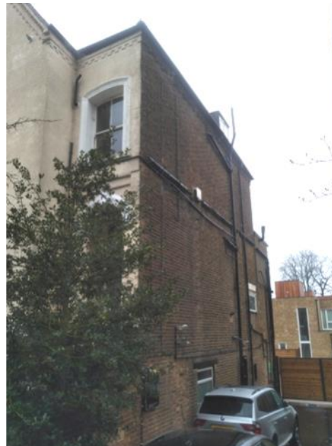
Figure 5.10: Showing the north-eastern elevation of No. 18. This also shows the entrance bay of the house.
