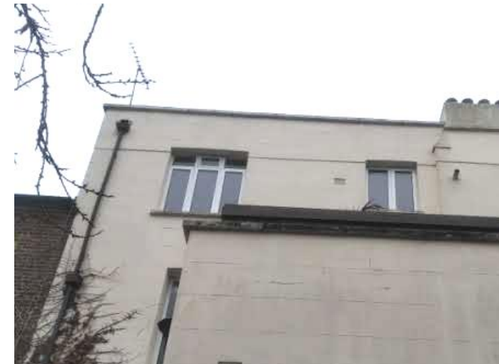
Figure 5.38: Showing the second floor rear of No. 17.
