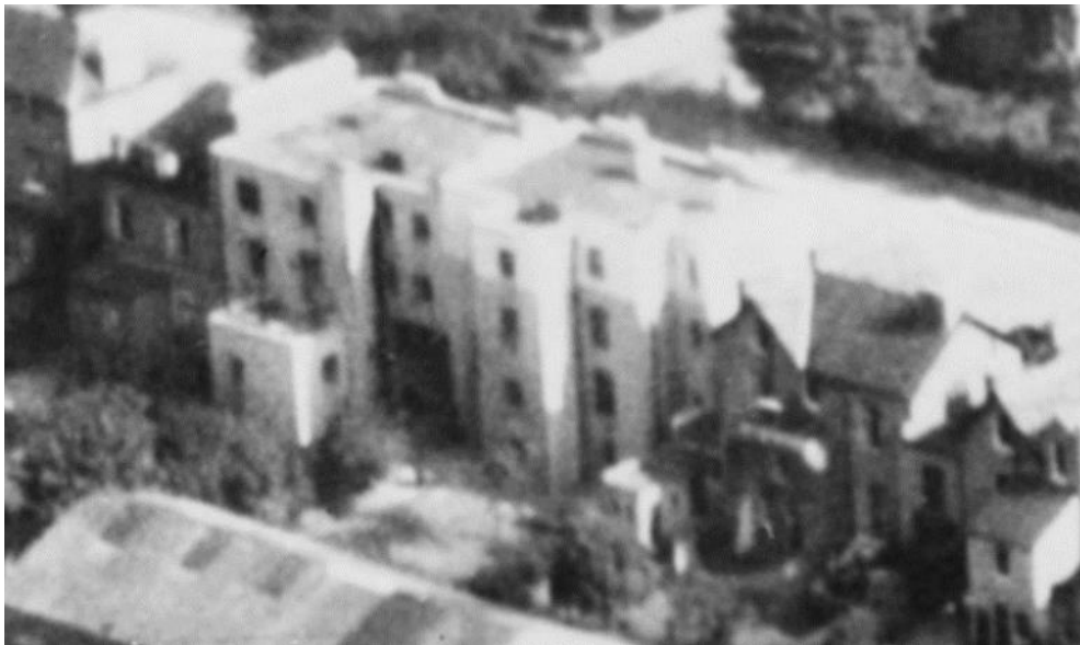
Figure 5.6: Showing the rear elevation in 1938 (Source: Britain from Above). Note there are no flat faux gables along the parapet line on the rear elevation of the building at this time.
