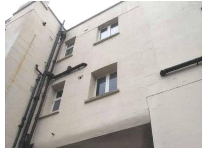
Figure 5.32: Showing the rear elevation of the Infill Extension.
