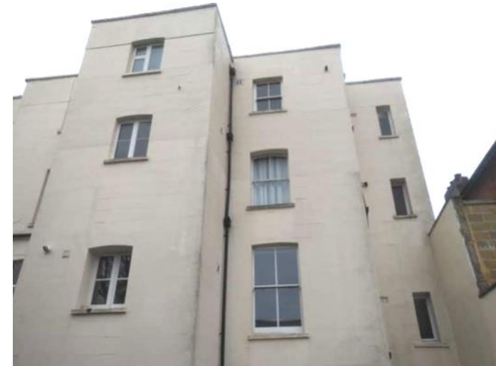
Figure 5.29: Showing the western side of the rear elevation at raised ground floor to second floor levels.
