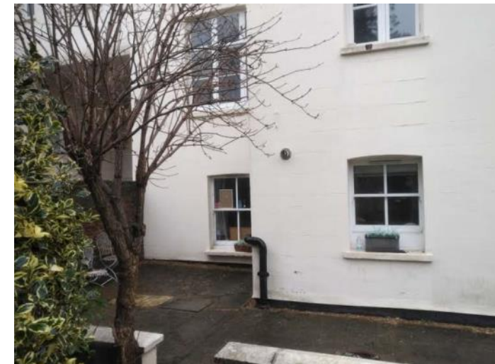
Figure 5.28: Showing the eastern side of the rear elevation at lower ground and raised ground floor level.
