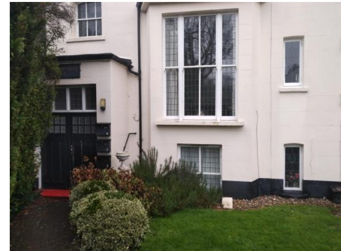
Figure 5.14: Showing the front porch.
