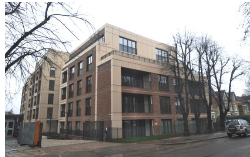
Figure 6.10: New 5-storey scheme adjoining the former Town Hall.
