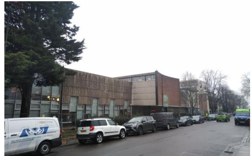
Figure 6.8: Hornsey Library on Haringey Park.
