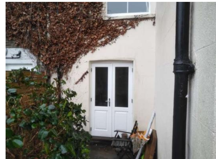
Figure 5.34: Showing the rear elevation of the main building at lower ground floor level.
