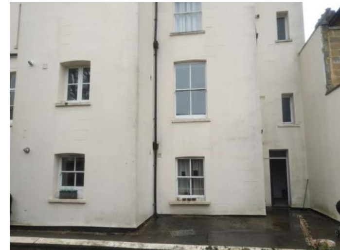
Figure 5.27: Showing the western side of the rear elevation at lower ground and raised ground floor level.
