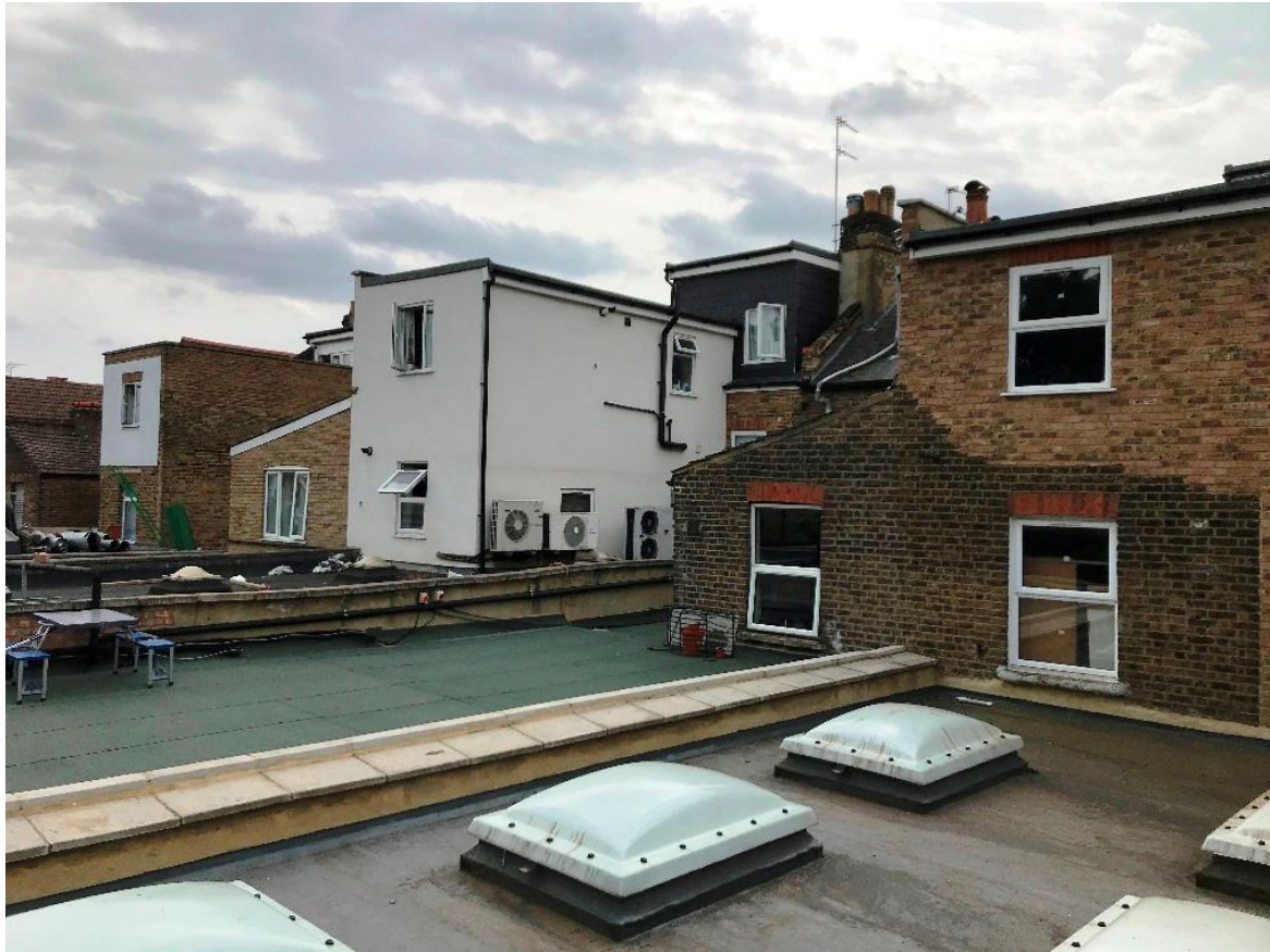
EXISTING ROOF VIEW
