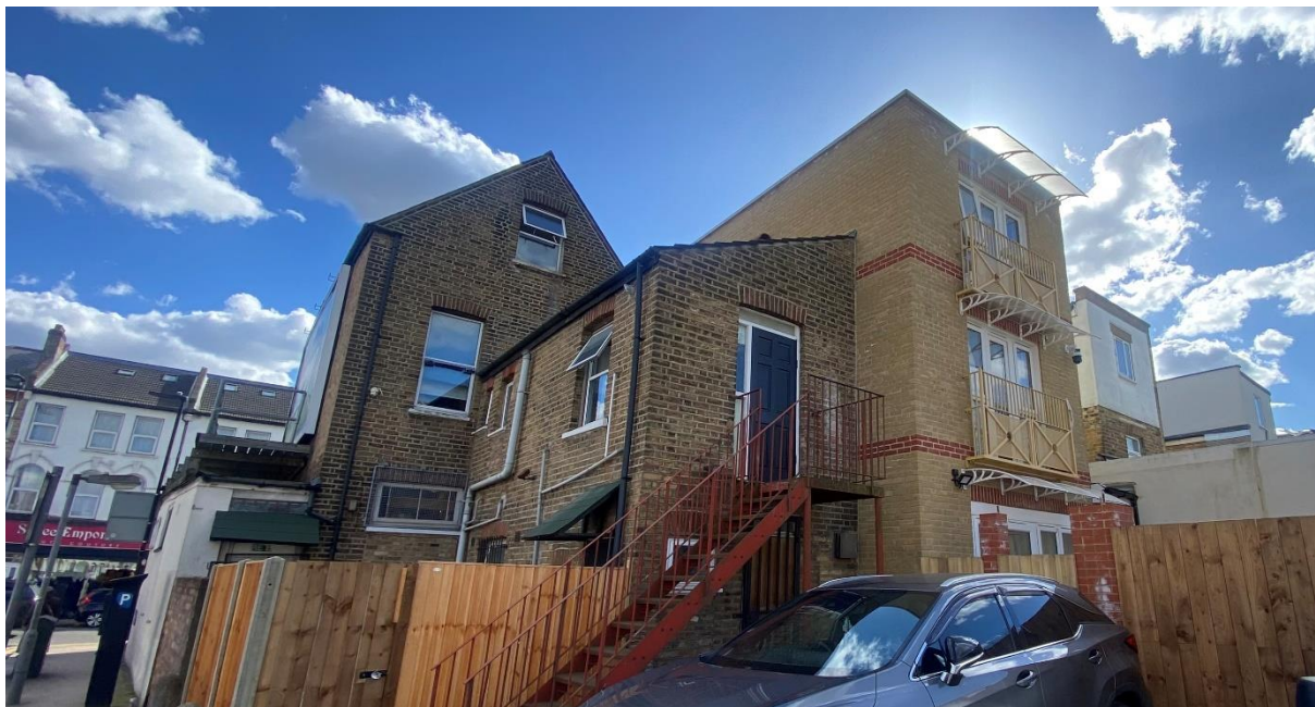
RECENT REAR EXTENSION TO NO 62
