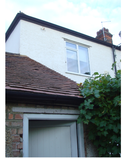
Fig 11. Rear garage roof &amp; main house
