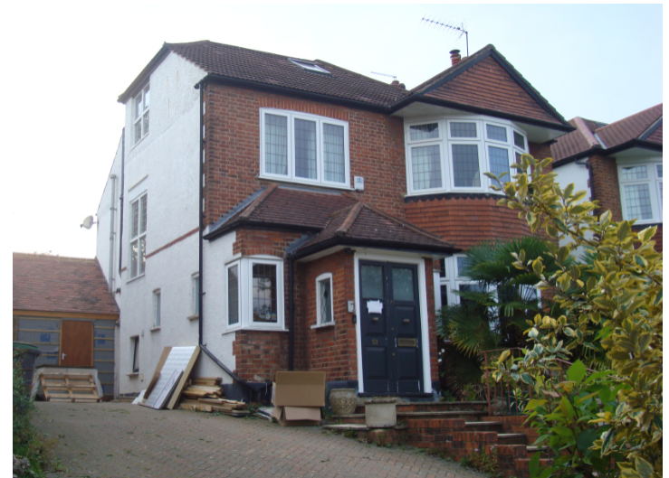
Fig 13. Front &amp; side view of number 59 Grove Avenue
