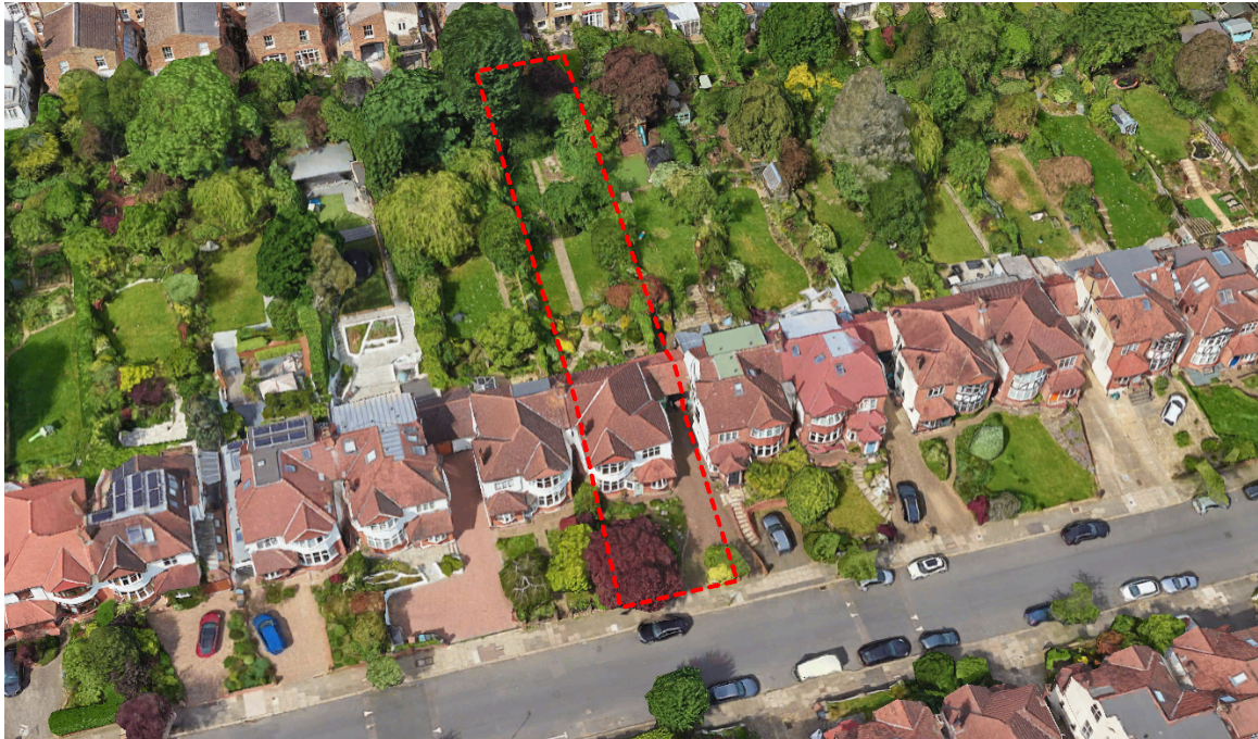
Fig 1. Aerial view along the East side of Grove Avenue.
