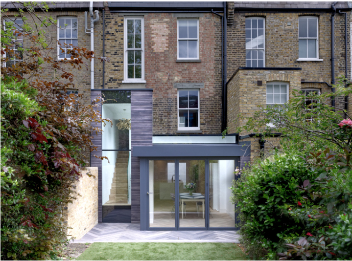
Fig 2. Rear view of Brookesley Street, E3 - Conservation Area, Tower Hamlets
