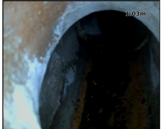
Defective Connection
