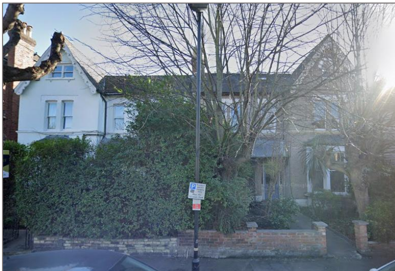
Front image of the semi-detached villa –No. 84 is the right-hand side.
