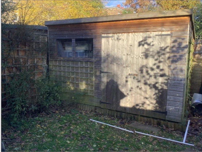
Existing shed which will be demolished to make way for the new garden room.
