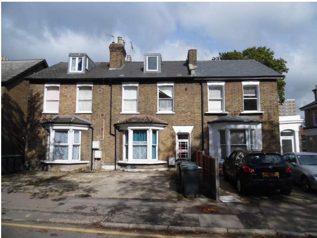
Front View from Trinity Road
