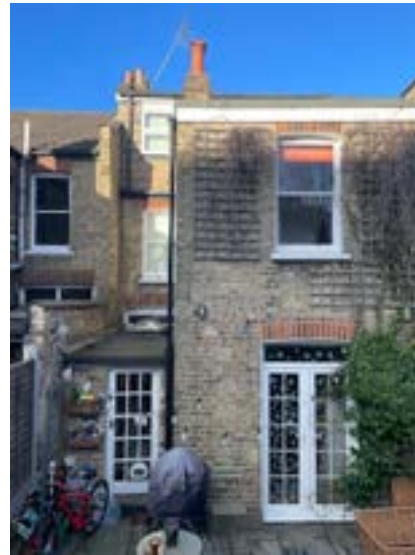
view of rear elevation
