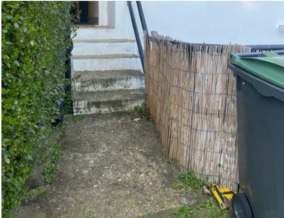
Existing entrance floor finish and railing along the entrance steps.
