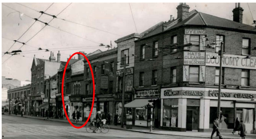
1950's Shopfront (highlighted in red).
