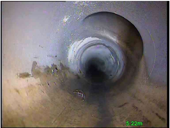
2, 00:00:24, 5.22 m Junction at 2 o'clock, 100mm dia
