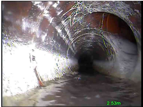
2, 00:00:17, 2.53 m Junction at 2 o'clock, 100mm dia
