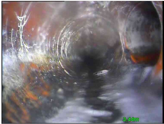
3, 00:01:53, 3.44 m Junction at 3 o'clock, 100mm dia
