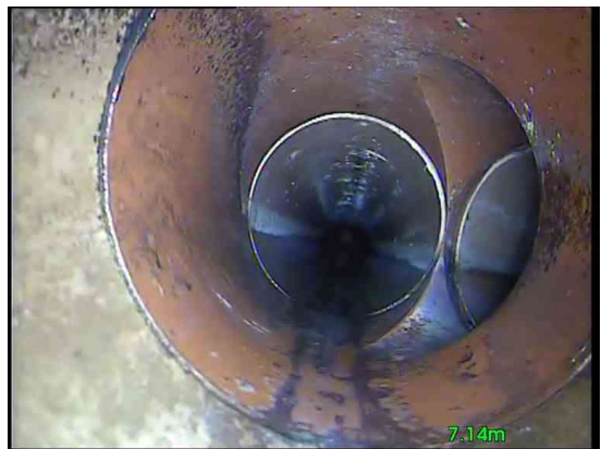
4, 00:00:31, 7.14 m Junction at 3 o'clock, 100mm dia
