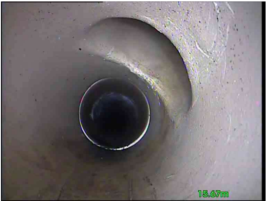
5, 00:01:01, 15.67 m Junction at 2 o'clock, 100mm dia
