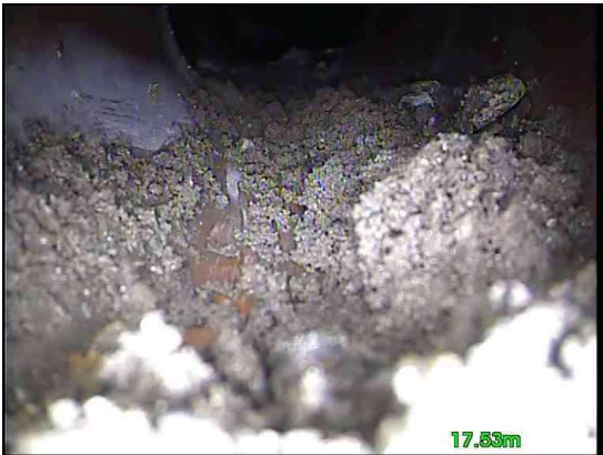
7, 00:01:28, 17.53 m Finish node, manhole, reference: MH7 reached
