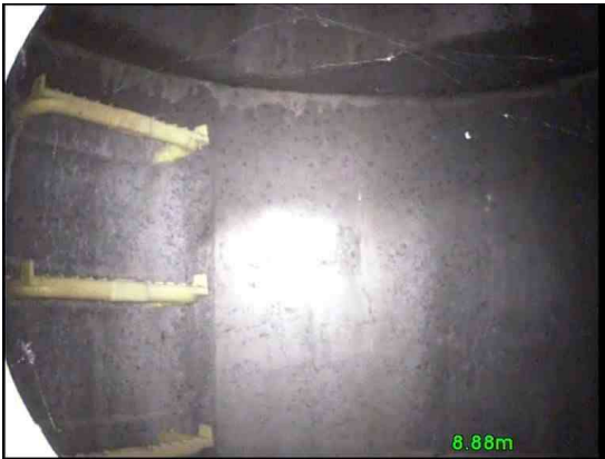
5, 00:00:52, 8.88 m Finish node, manhole, reference: MH26 reached
