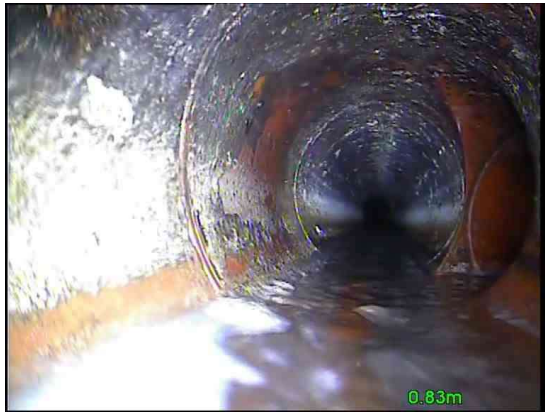
1, 00:00:10, 0.83 m Junction at 3 o'clock, 100mm dia
