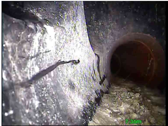
5, 00:00:30, 7.36 m Finish node, manhole, reference: MH27 reached
