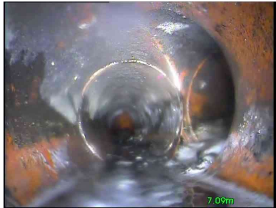
6, 00:01:31, 7.09 m Junction at 9 o'clock, 100mm dia
