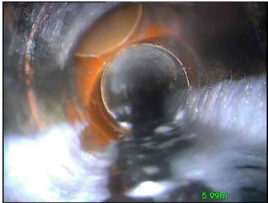
5, 00:01:37, 5.99 m Junction at 10 o'clock, 100mm dia
