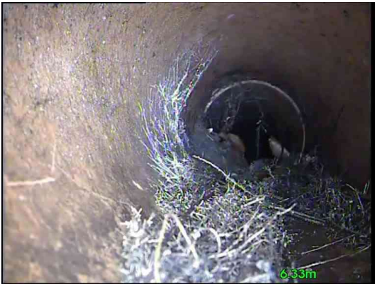
9, 00:00:55, 6.33 m Roots, mass, 35% cross-sectional area loss, change
