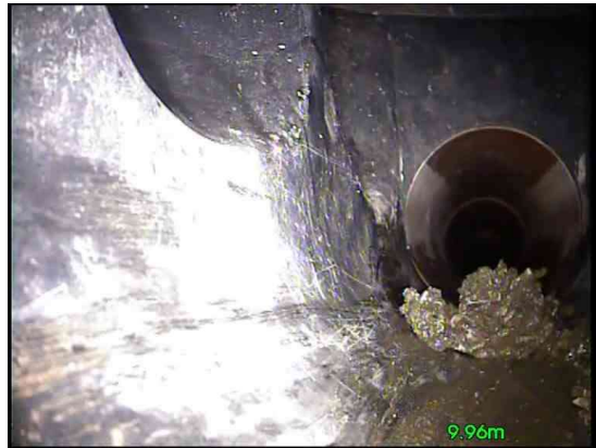
6, 00:00:46, 9.96 m Finish node, manhole, reference: MH35 reached
