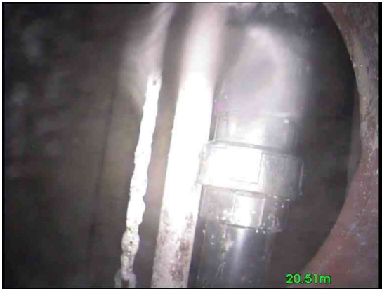
6, 00:01:50, 20.51 m Finish node, manhole, reference: MH38 (Pumping Station) reached
