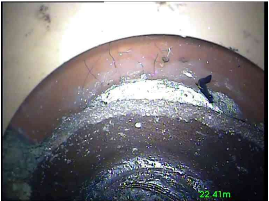
24, 00:02:38, 22.41 m Finish node, gully, reference: RWP reached
