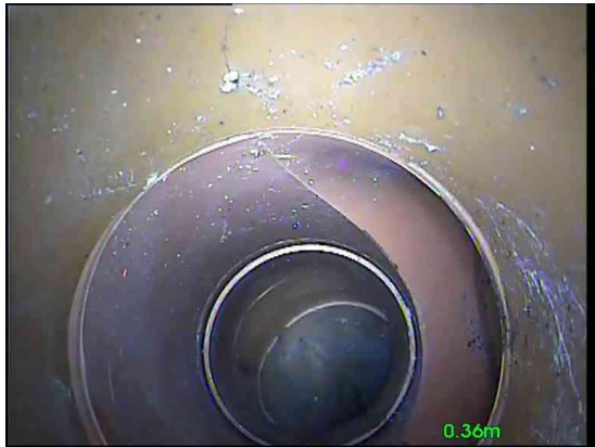
1, 00:00:09, 0.36 m Junction at 3 o'clock, 100mm dia
