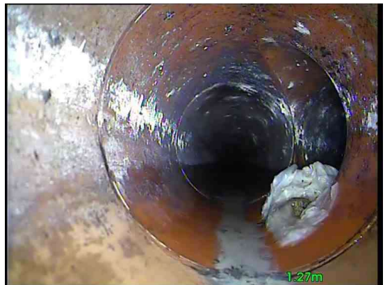
2, 00:00:08, 1.27 m Junction at 3 o'clock, 100mm dia
