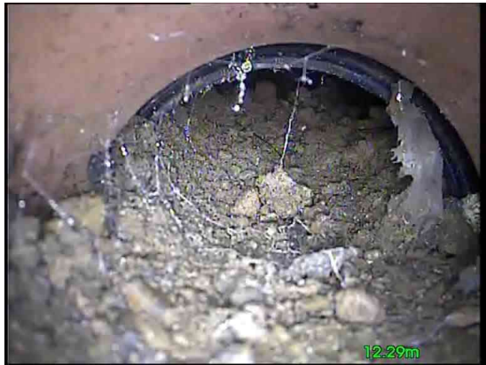
10, 00:00:53, 12.29 m Finish node, rodding eye, reference: RE reached
