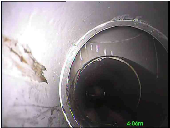
6, 00:00:34, 4.06 m Junction at 11 o'clock, 100mm dia
