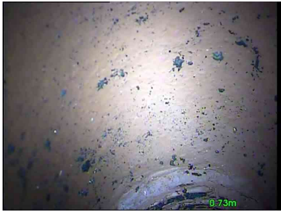
3, 00:00:11, 0.73 m Finish node, gully, reference: RWP reached
