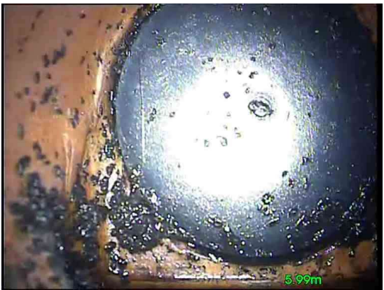
6, 00:00:42, 5.99 m Finish node, gully, reference: RWP reached
