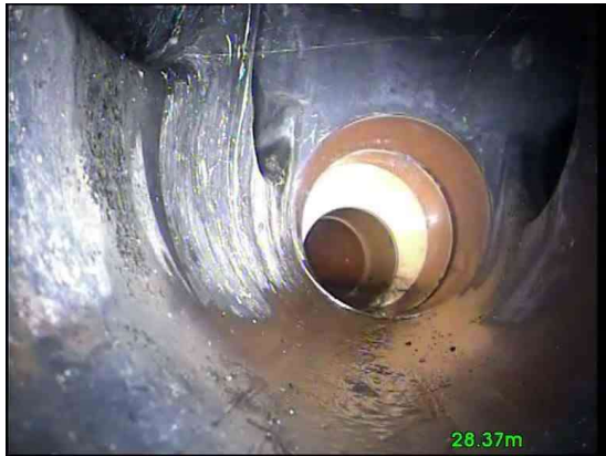
9, 00:01:34, 28.37 m Finish node, manhole, reference: MH11 UTL reached
