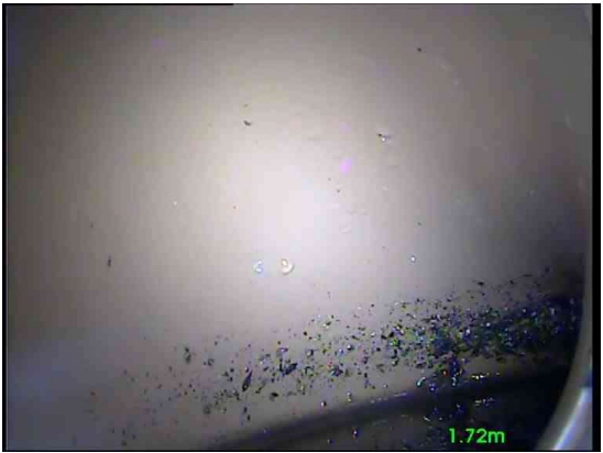
4, 00:00:19, 1.72 m Finish node, gully, reference: RWP reached
