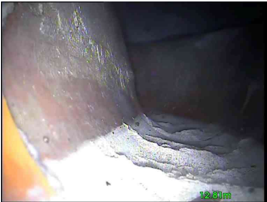
11, 00:01:01, 12.81 m Finish node, manhole, reference: MH31 UTL reached
