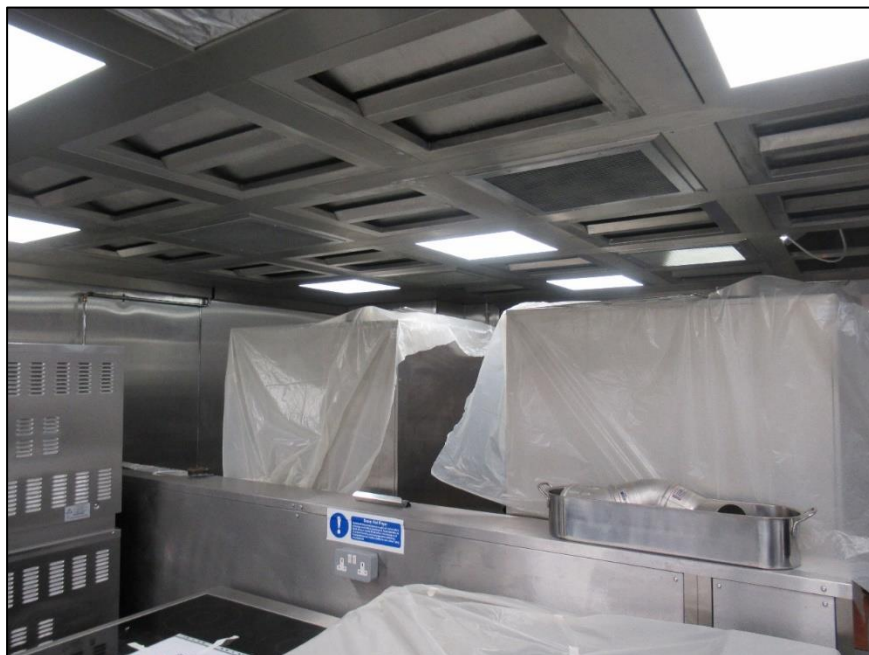
Figure 12: Basement Level 1 Kitchen (A)
