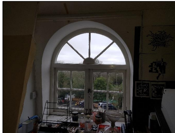
Figure 53: Level 3 Window (B)
