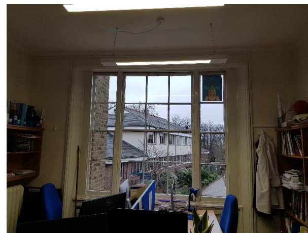
Figure 36: Level 1 Windows (E)
