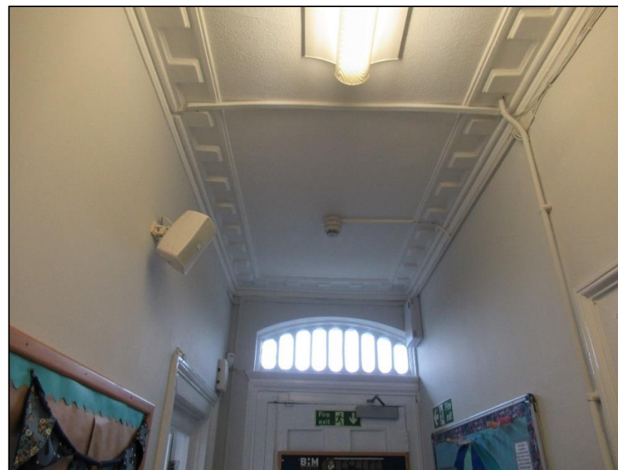
Figure 22: Room 4 – Ceiling Cornice and Fanlight Above Doorway
