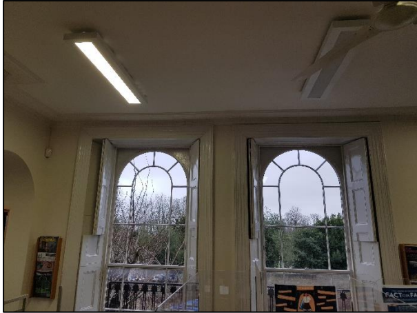
Figure 32: Level 1 Windows (A)
