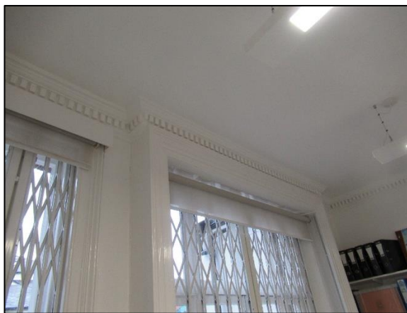
Figure 16: Room 1 - Cornice Above Windows
