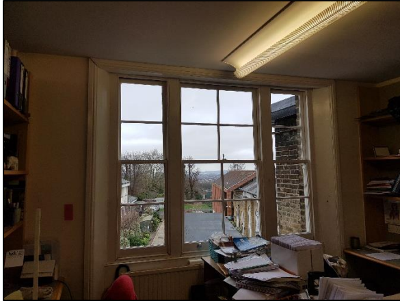
Figure 44: Level 2 Window (A)
