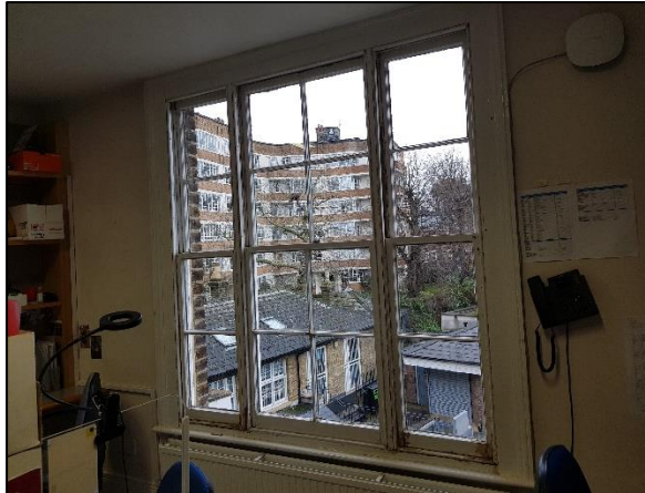
Figure 45: Level 2 Window (B)
