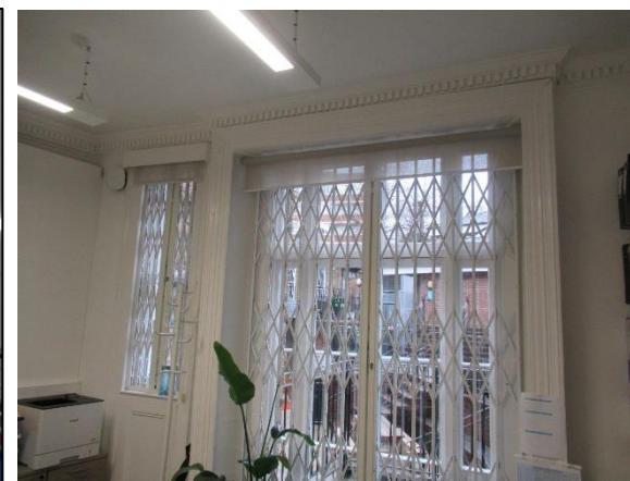
Figure 17: Room 1 – Surviving Cornice and Frame
