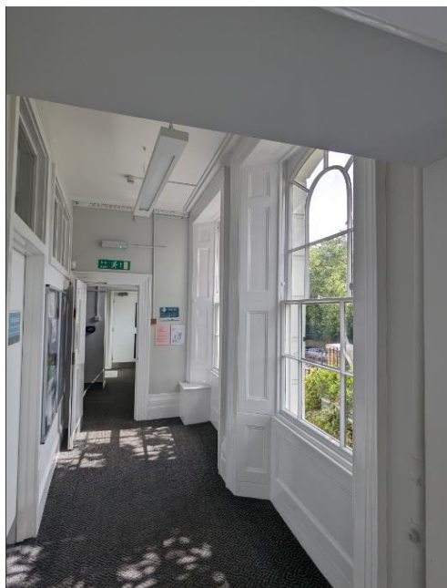
Figure 27: Window Bays (A)
