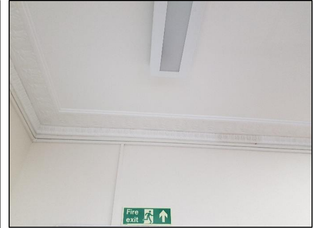
Figure 40: Level 1 Cornice (C)
