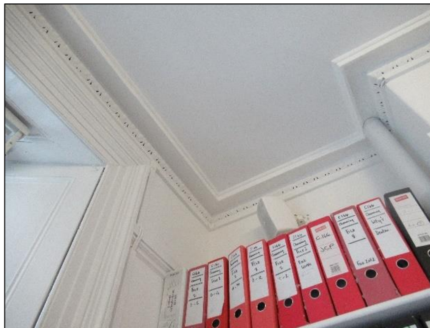
Figure 24: Painted Over Cornice (B)
