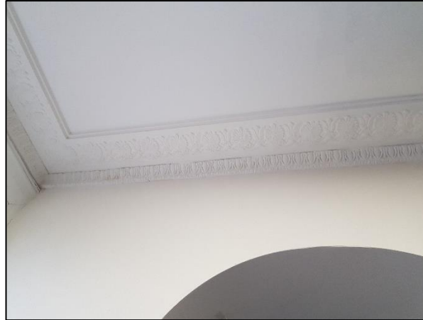
Figure 39: Level 1 Cornice (B)
