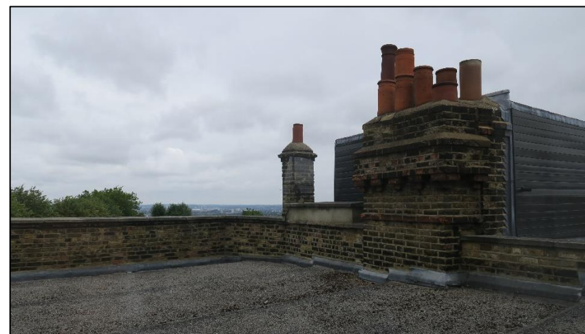
Figure 61: Existing Chimney to be Removed
