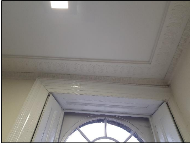
Figure 38: Level 1 Cornice (A)
