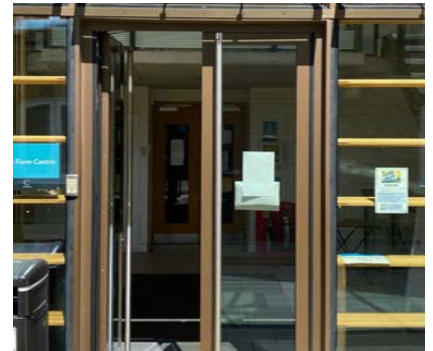
Fig. 18. Coated aluminium doors
