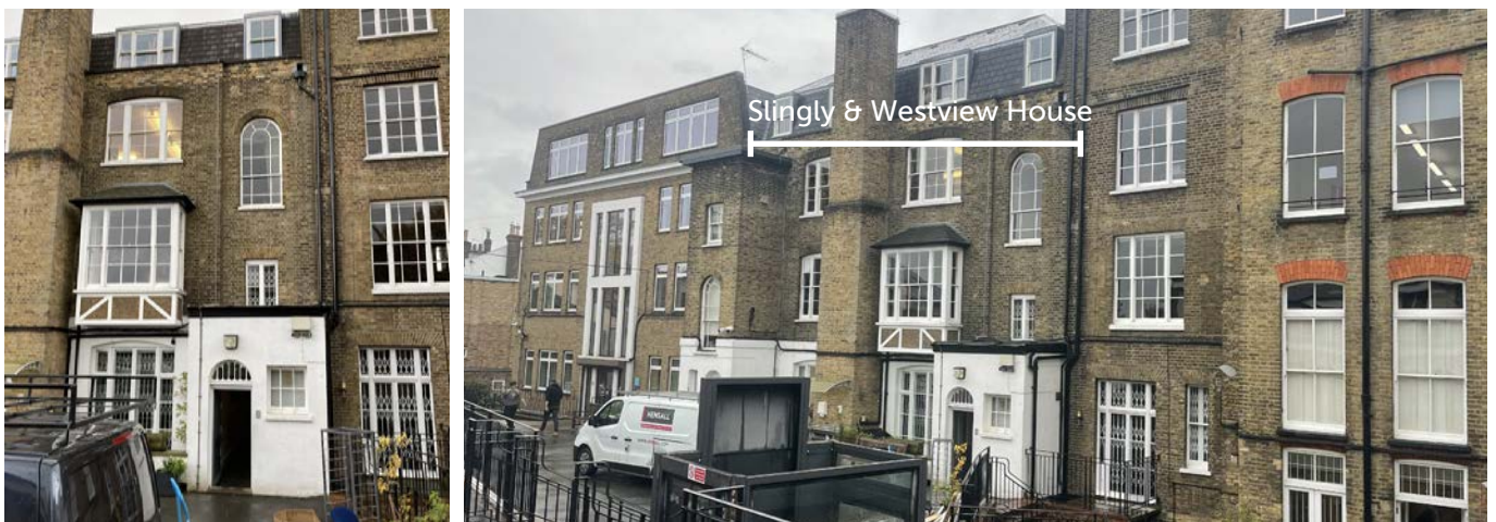
Fig. 8 and 9 - Rear of Slingly House and Main School Building
