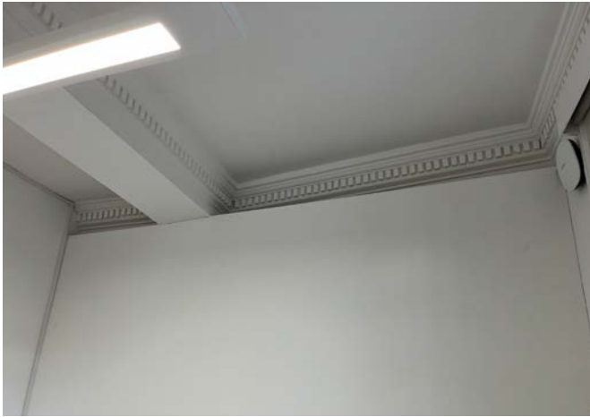
Fig. 16 - Level 0 - Decorative beam and cornice concealed by modern partition
