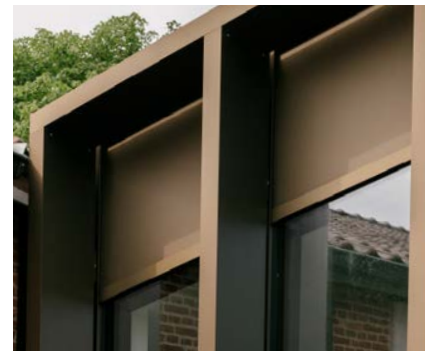
Fig. 20. Coated aluminium metal fins
