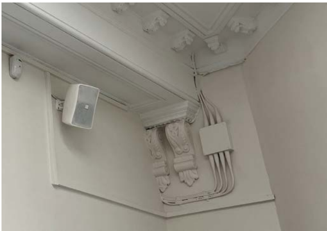
Fig. 18 - Level 0.5 - Decorative beam and corbel concealed by modern partition
