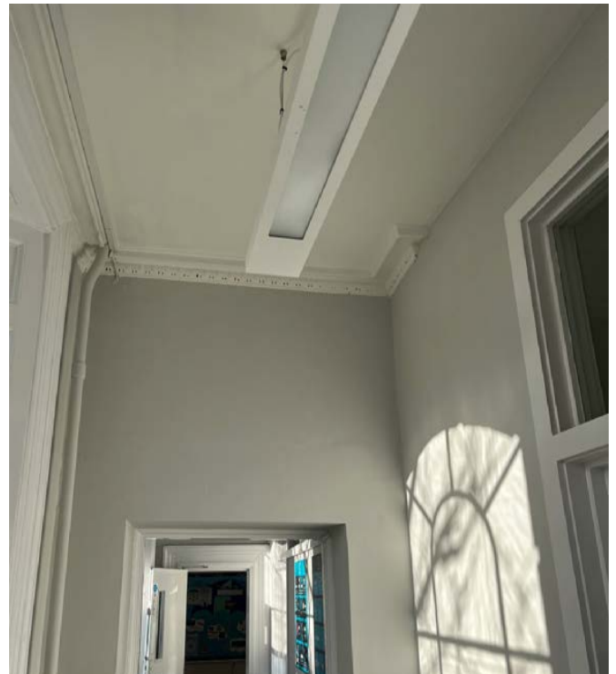
Fig. 19 - Level 0 - Decorative cornice concealed by modern partition
