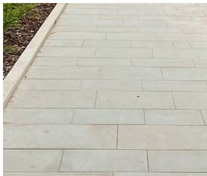
Fig. 21. Permeable paving slabs
