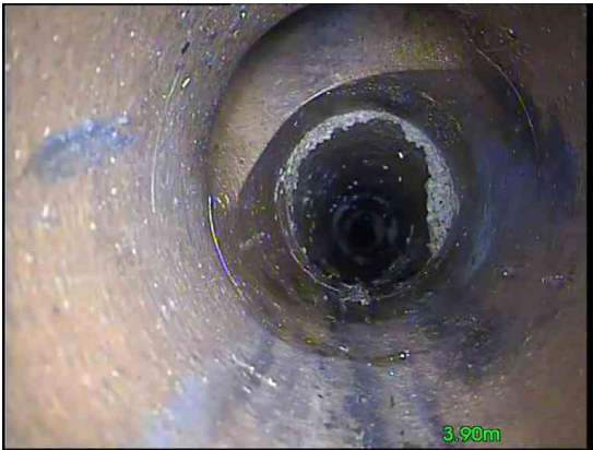
5, 00:00:30, 3.90 m Junction at 11 o'clock, 100mm dia
