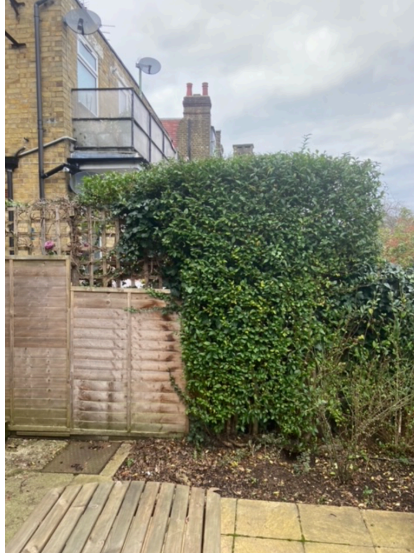
Boundary timber fence to n° 54 (2.47m, from floor finish to top of timber)
