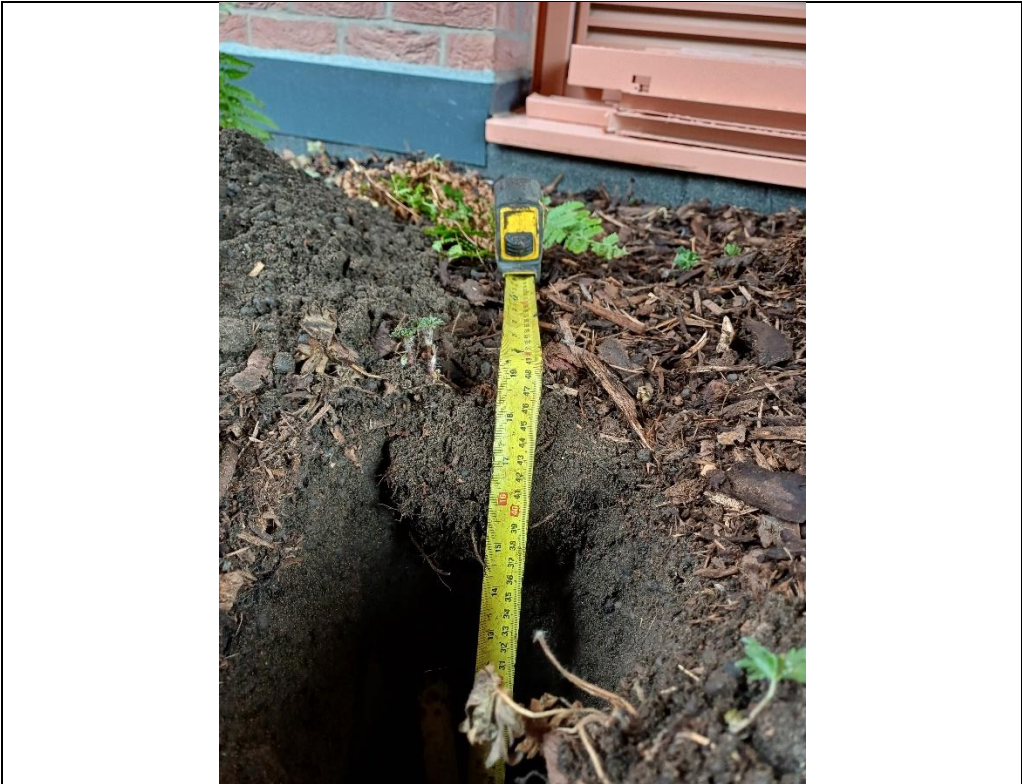
Plate 4: Podium level planter – clean cover thickness.
