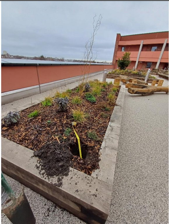
Plate 5: Roof level planter – general view.
