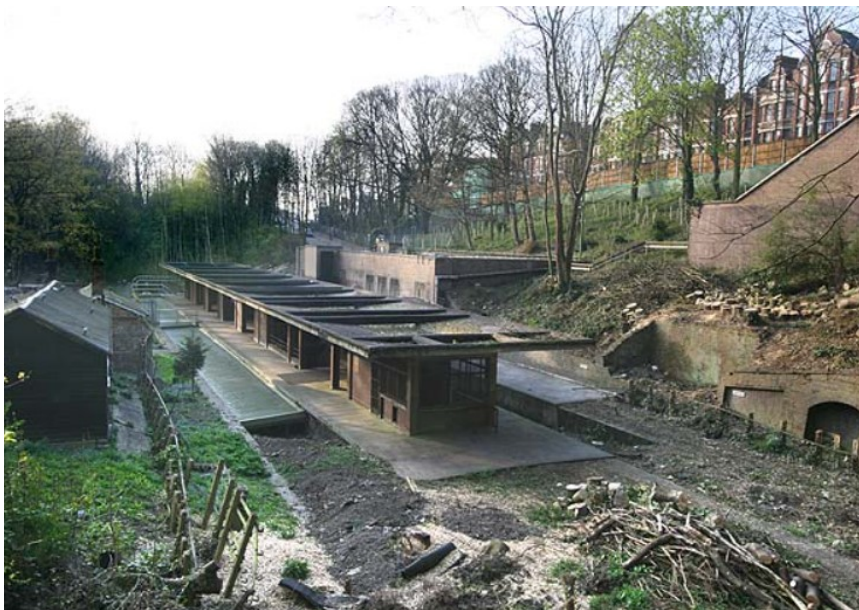
Picture 2 – Highgate Station looking East, circa 2007. The track beds are covered in corrugated plastic to mitigate issues with the Northern Line below. The original 1867 building in question can be seen on the left-hand side
