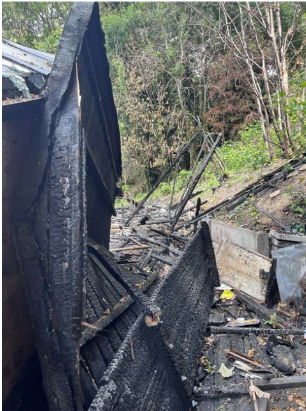
Photo 17 – Rear Elevation showing remains of razed timber building – note PC retaining structure supporting raised bank to public footpath
