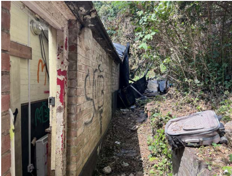
Photo 15 - Rear (NE) Elevation leading to remains of razed timber building
