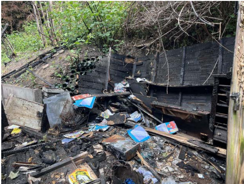
Photo 18 - Rear Elevation showing remains of razed timber building
