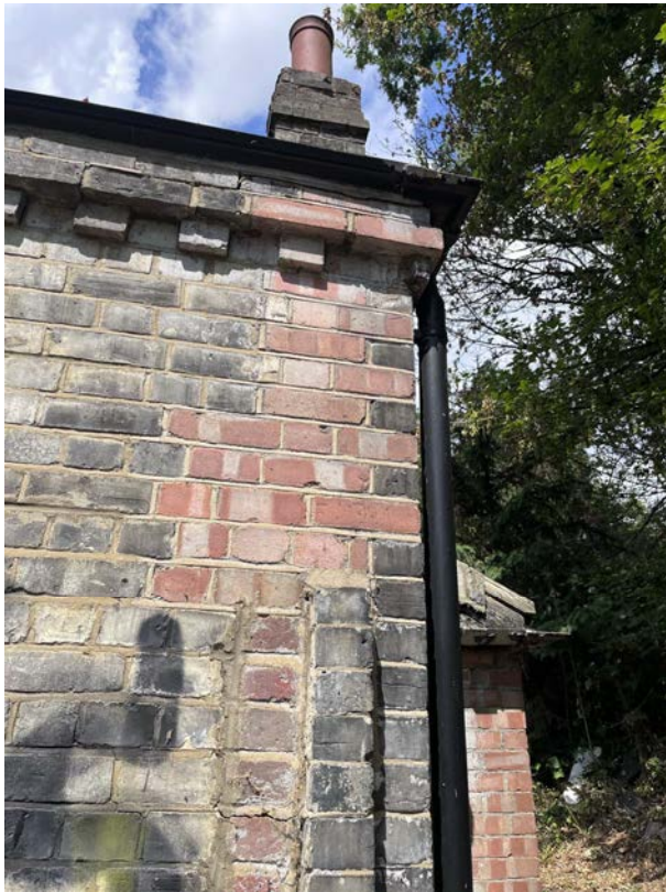
Photo 13 - Side Elevation (SE) showing rebuilt structure at corner with Rear
