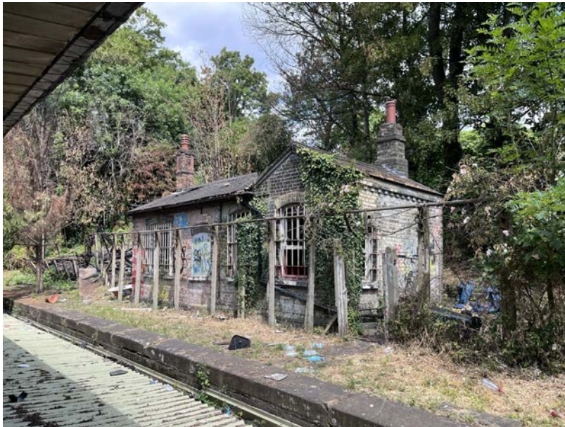
Photo 1 – Front Elevation facing redundant track
