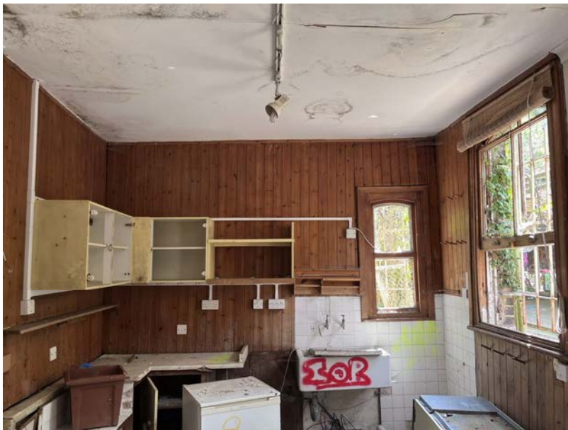
Photo 22 – Internal kitchen area
