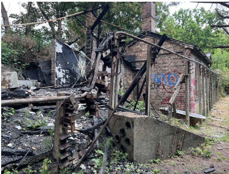
Photo 4 – Side (NW) Elevation showing area of razed Timber Building
