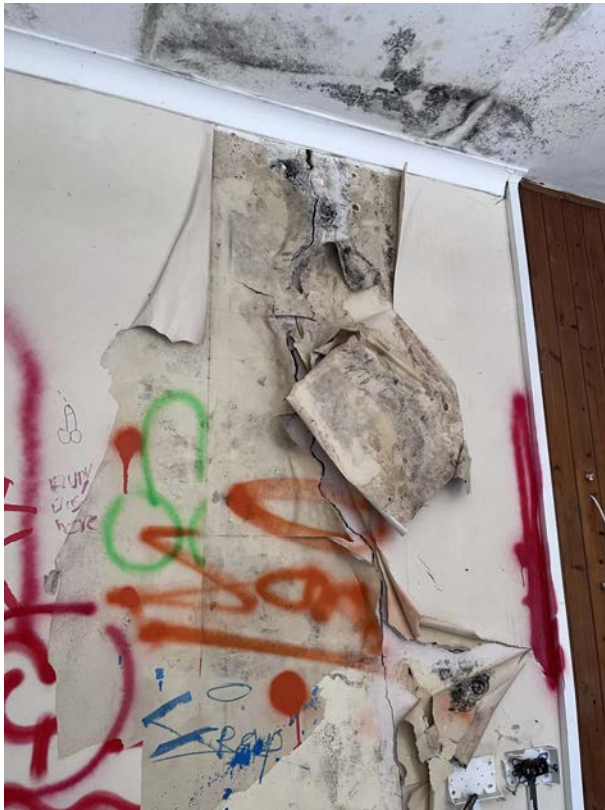
Photo 23 – Internal kitchen area showing large vertical crack to load bearing wall
