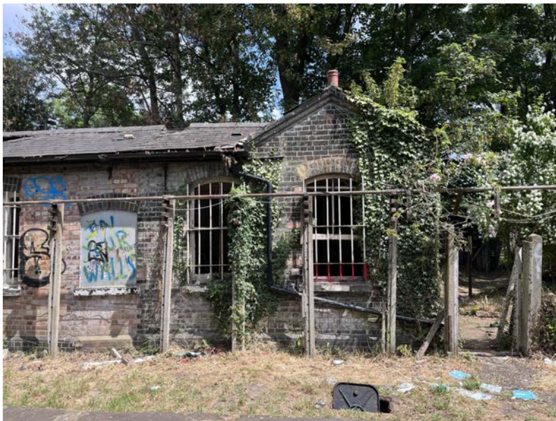
Photo 2 – Front Elevation RHS
