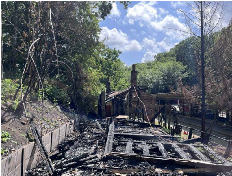
Photo 28 – Rear Elevation showing remains of razed timber building – note PC retaining structure supporting raised bank to public footpath
