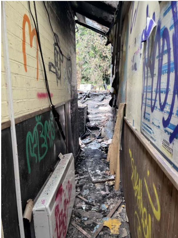
Photo 21 – Internal lean-to walkway to rear/remains of razed timber building
