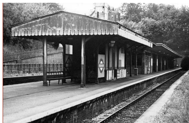
Figure 4: The 1939-41 rebuilt station structure at the far end, with the retained canopy and toilets in the foreground, photographed just after the Second World War © Photomatic Ltd
