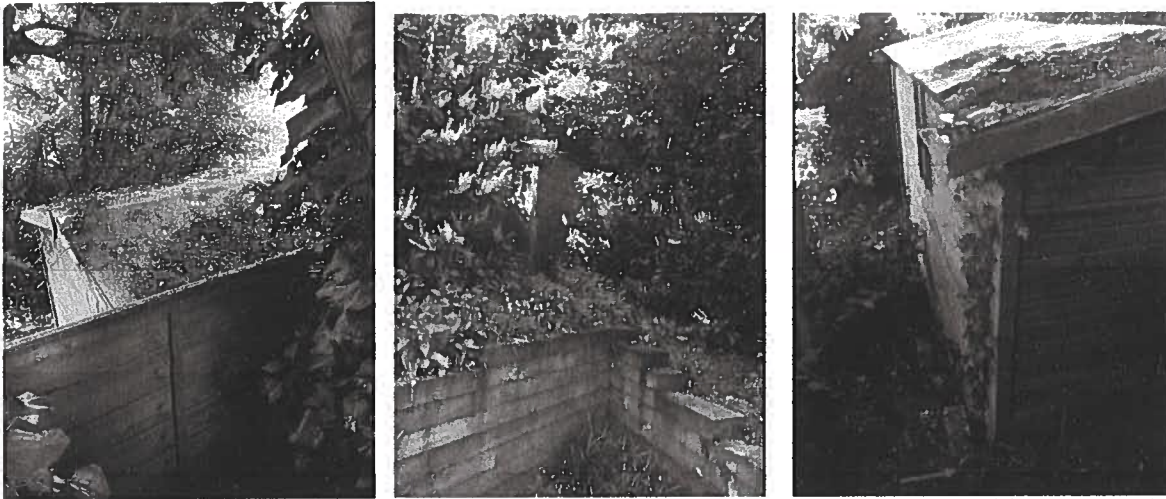
Figure 2 – Photographs showing the proximity of current shed to the boundary fence with 12 Kingsley Place
