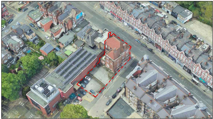
Aerial view of East Facing Facade
