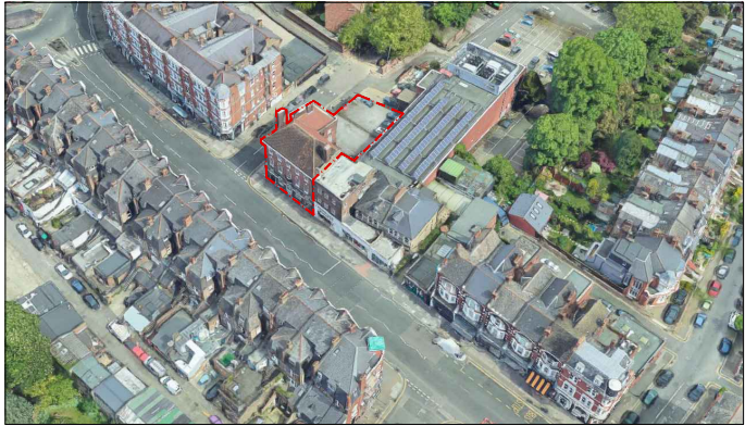
Aerial view of South Facing Facade
