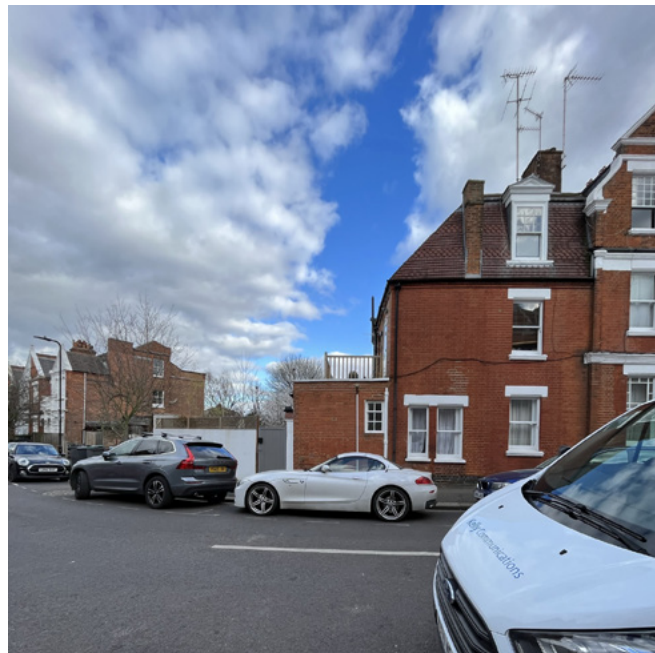
Photograph of existing building
