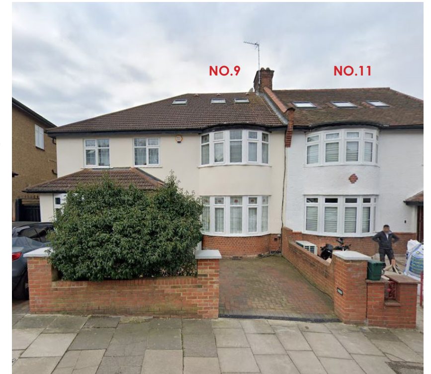
EXISTING BRICK PLINTH - FRONT ELEVATION
