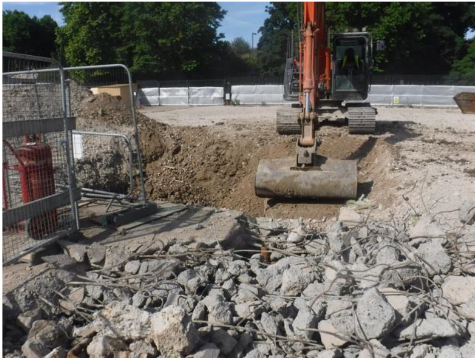
Extended excavation northerly below Tank 3.
