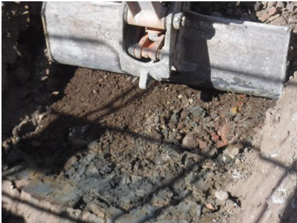
London Clay reached at approximately 3.10m Validation sample Base West 3.10m.
