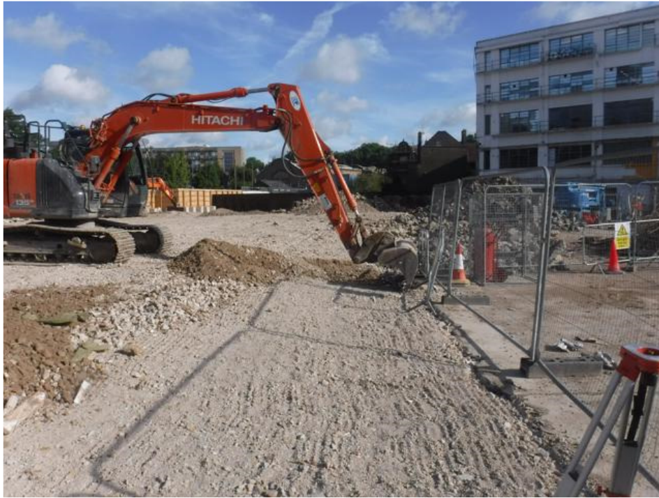
Looking northerly – excavation commenced above Tank 1.
