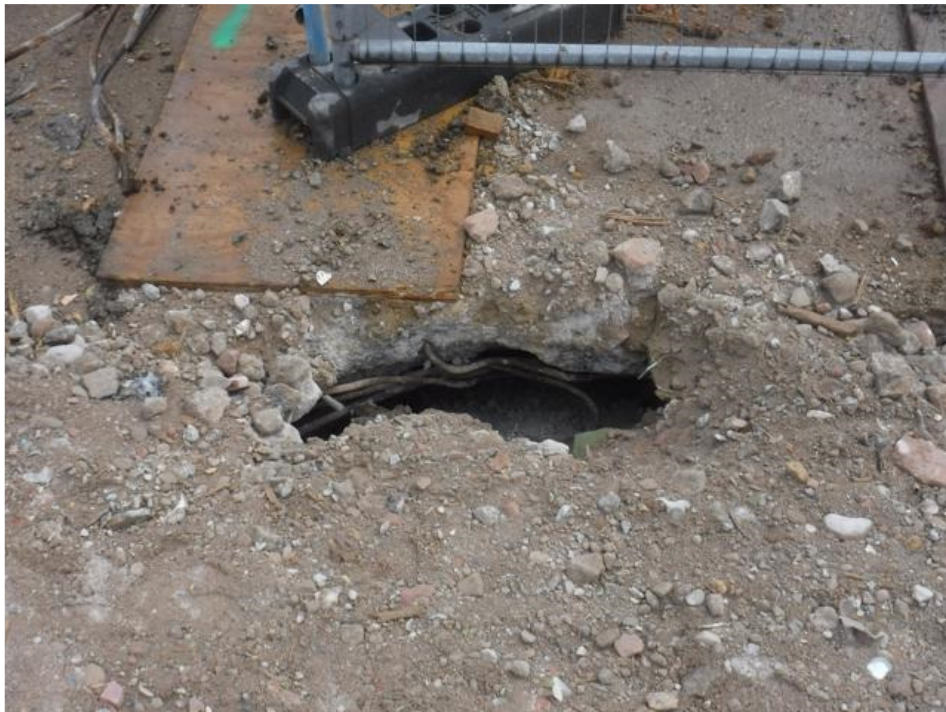
Tank 4 remains in-situ.
