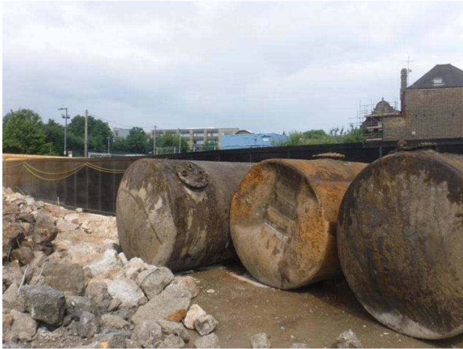
28 June 2022 – three exhumed USTs.
