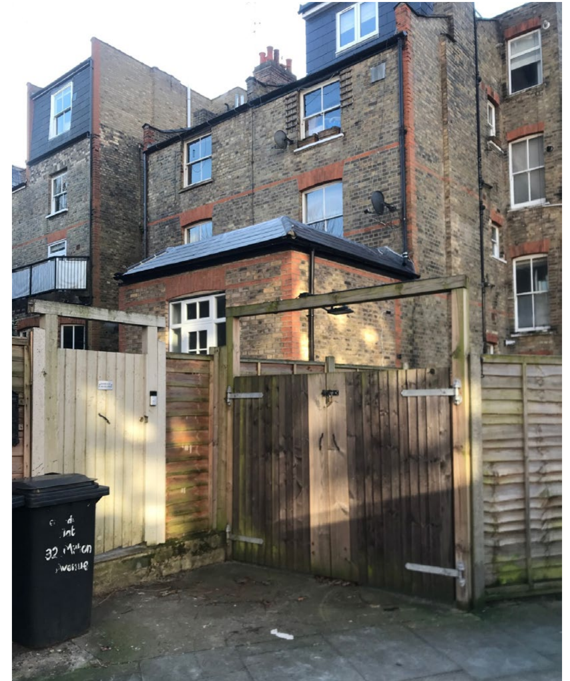
5.2 The current street view of the Garden Flat at 32 Milton Avenue.
