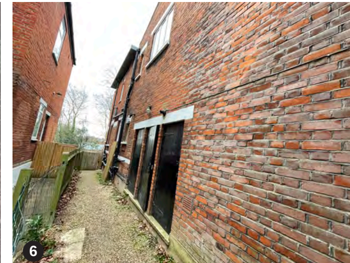
6 East facade path/ route
