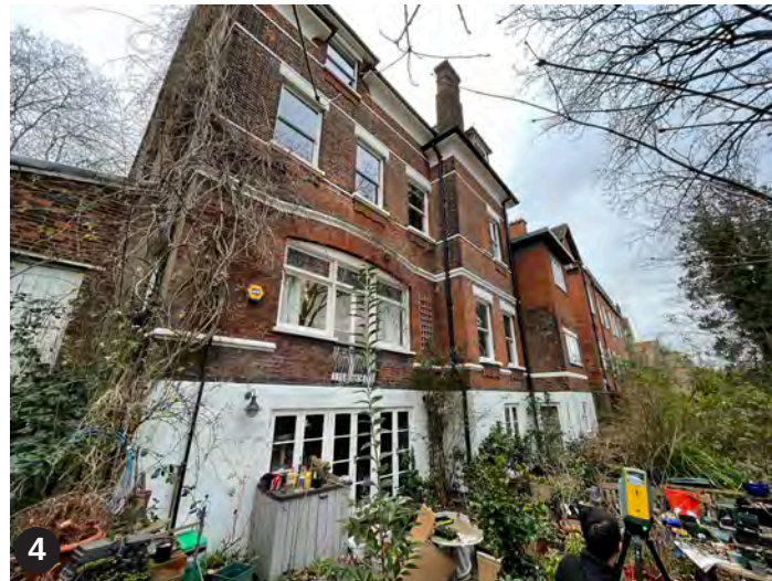
4 South Elevation/ Rear facade
