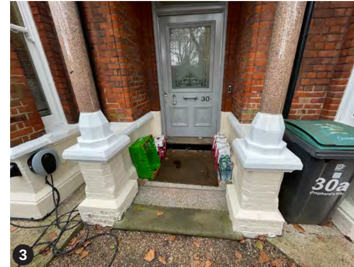
3 Entrance to 30 a ( Application Property)
