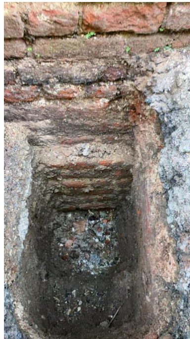
Image 10: The foundation of the wall
