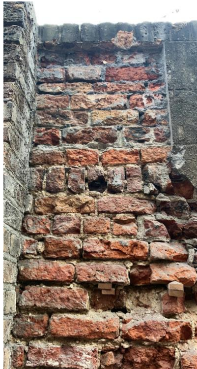
Image 2: The revealed condition of the core brickwork of the wall
