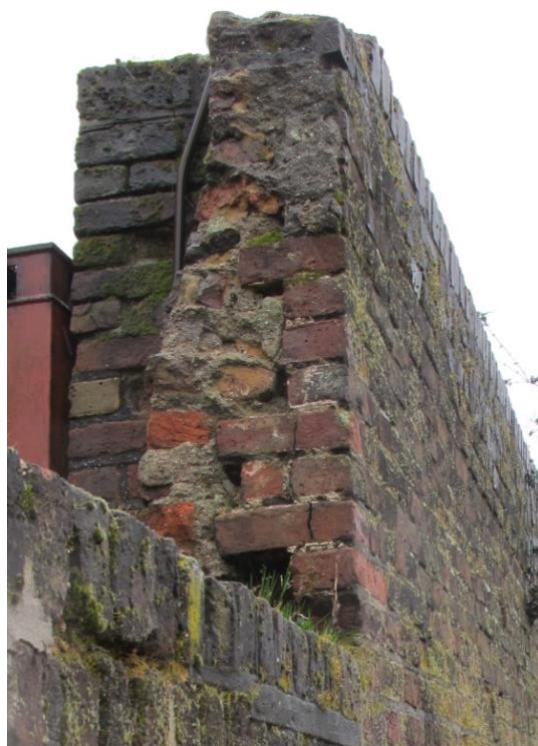
Image 3: Revealed battered profile
