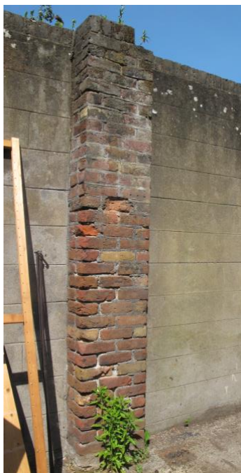
Image 4: Buttress piers along east elevation
