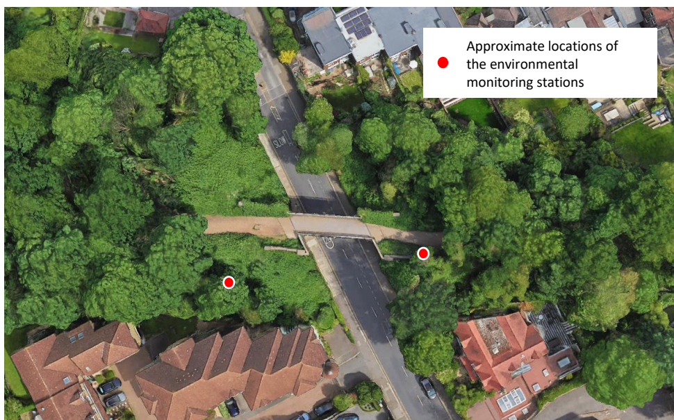
Figure 9: Approximate locations of the environmental stations which monitor noise, dust and vibration on Stanhope Road Bridge.
