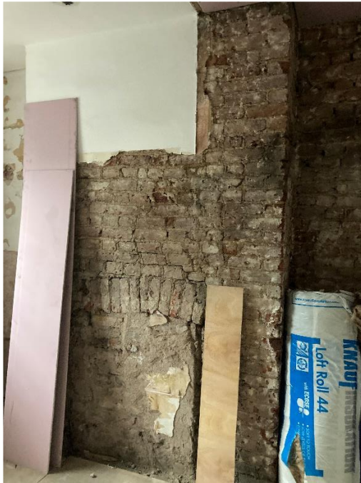
Above Left: Photo of 1 st floor bathroom wall with sanitaryware, stud partition wall and surrounding finishes removed. Above Right: With new plasterboard/ plastered finish to the wall.
