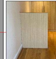
Non original dwarf wall
