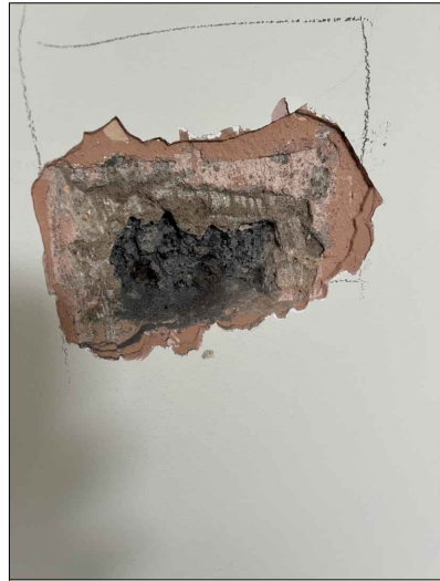
Modern block work
