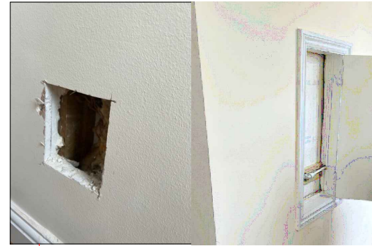
Modern Studwork partitions
