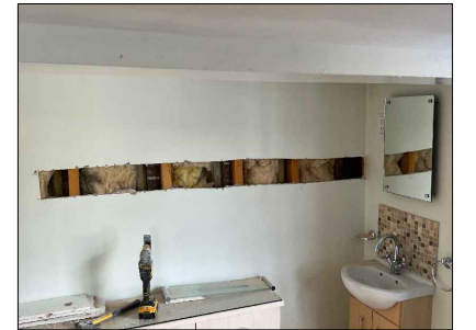
Doorway created by removing modern stud - no historic timbers to be removed. Further details in the Heritage Note.
