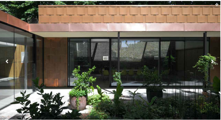
Frameless glazed walls to proposed extension
